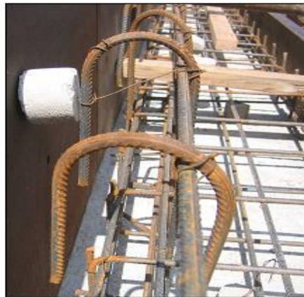
Fig.13 Correct cover blocks in place
