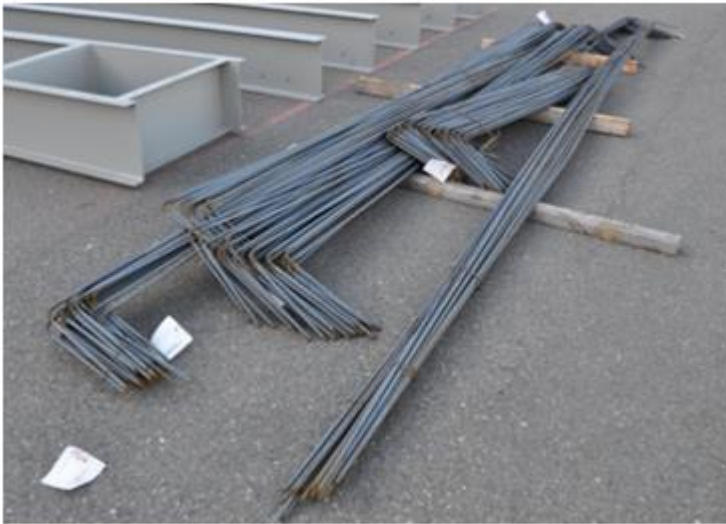
Fig.4 Example of cut & bent bar
