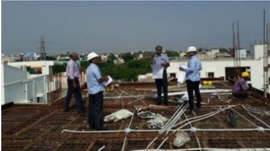
Fig. 2: Slab reinforcement checking
