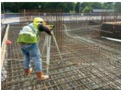
Fig. 1: Checking level of slab shuttering
