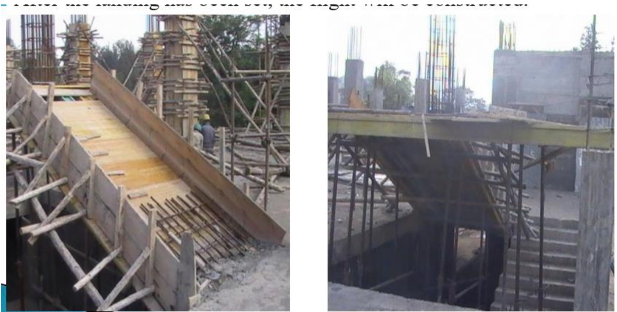
Fig.15. Timber stair formwork
