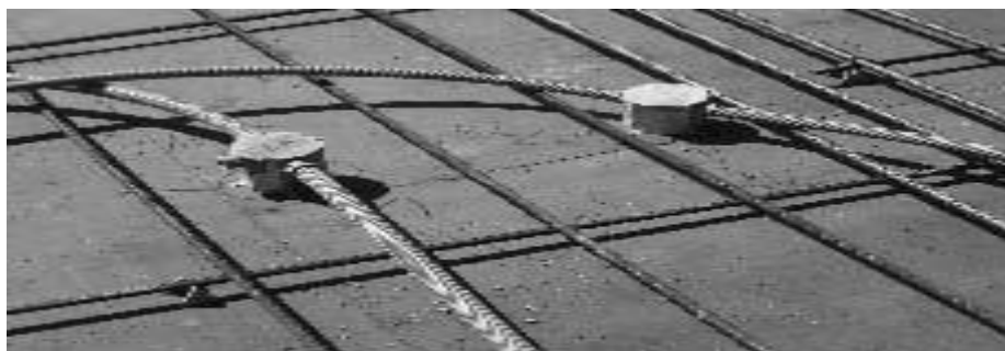
Fig 6.3. Junction boxes and conduit serve as sleeves.
