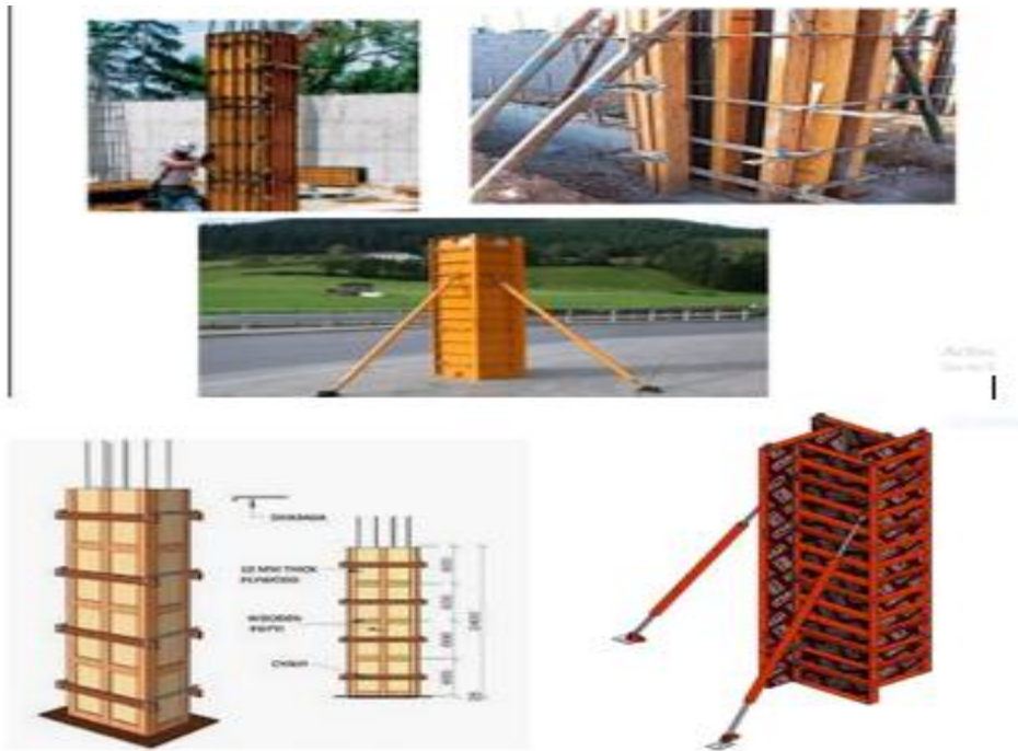
Fig 4 Formwork for column
