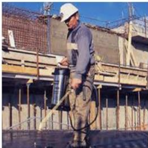
Fig 7.1 When applying releasing agents |
