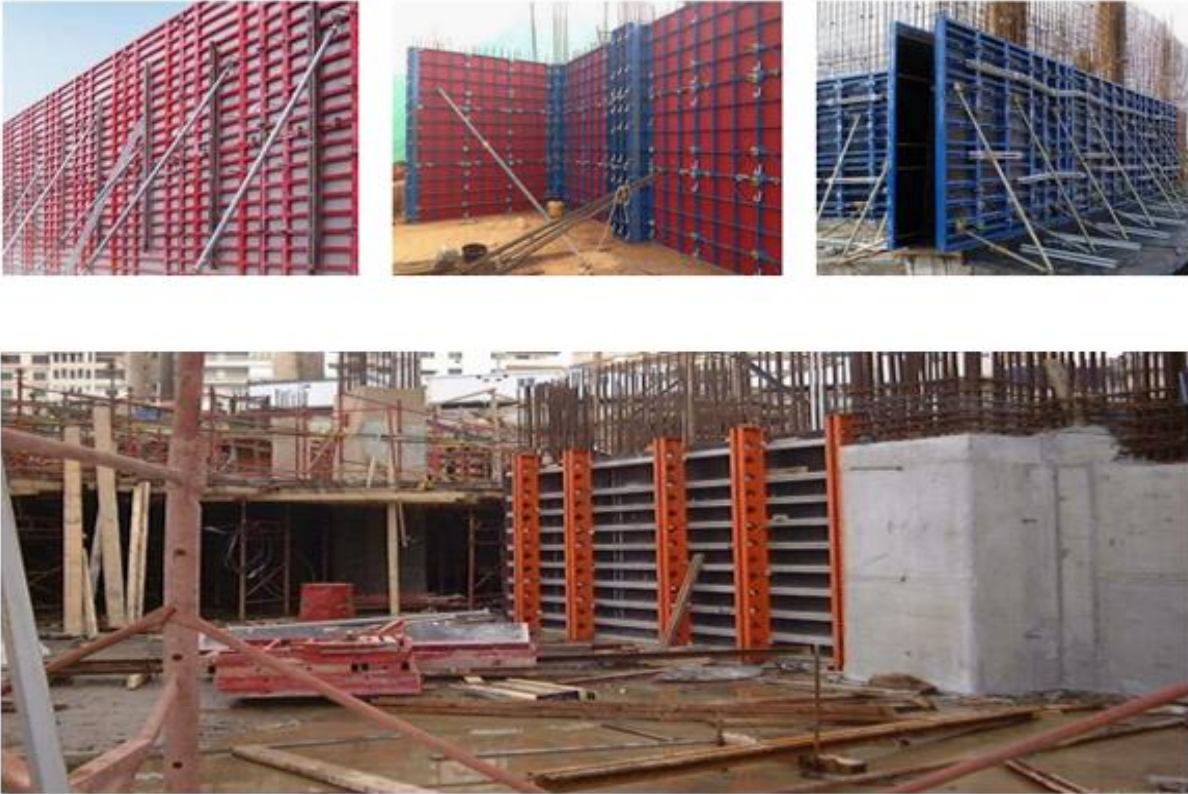
Fig 9. Metal formwork
