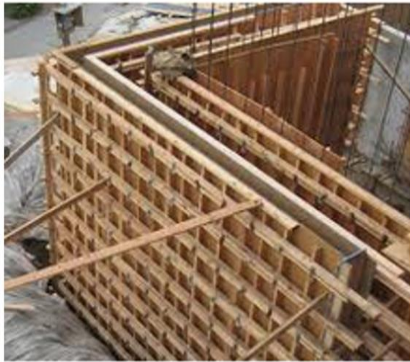
Fig 13 Wall Formwork
