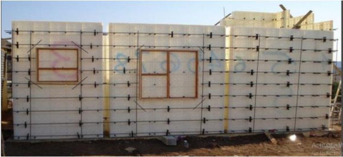
Fig 10 Plastic Formwork
