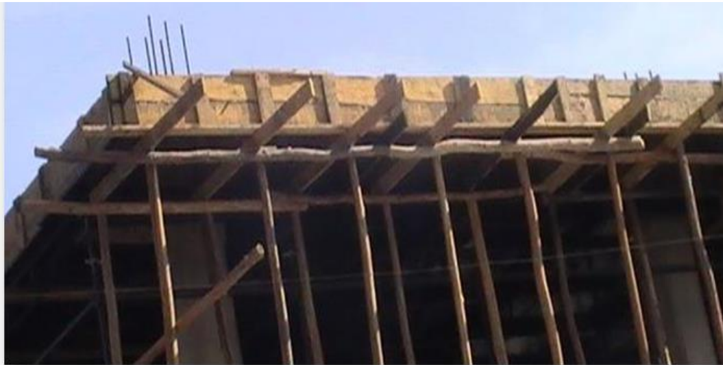
Beam and slab formwork
