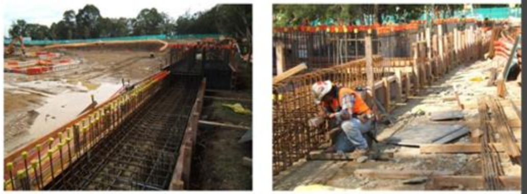
Fig 11.Beam Formwork
