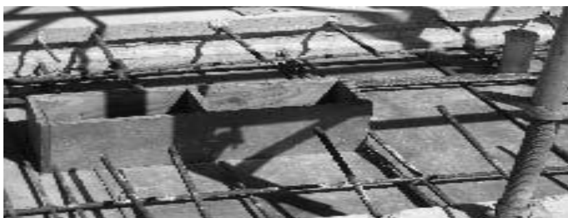
Fig 6.1 box-out sleeve on top of the slab form
