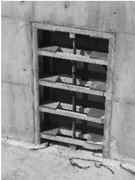
Fig 6.2. Buck used to create door opening
