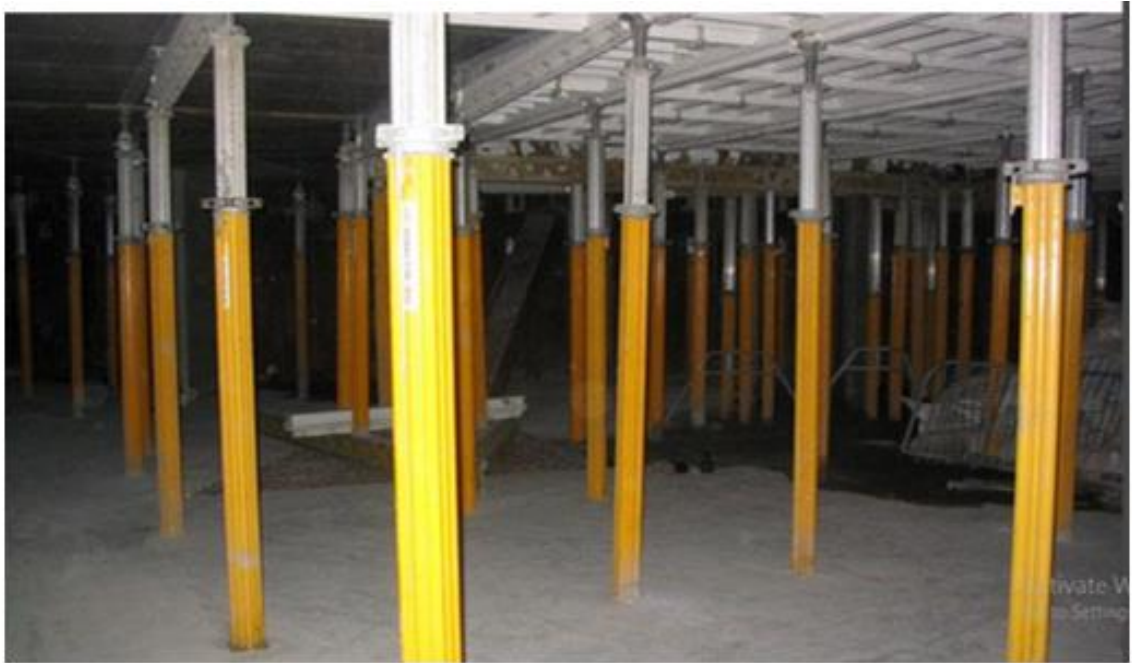
Fig 11 Steel slab formwork
