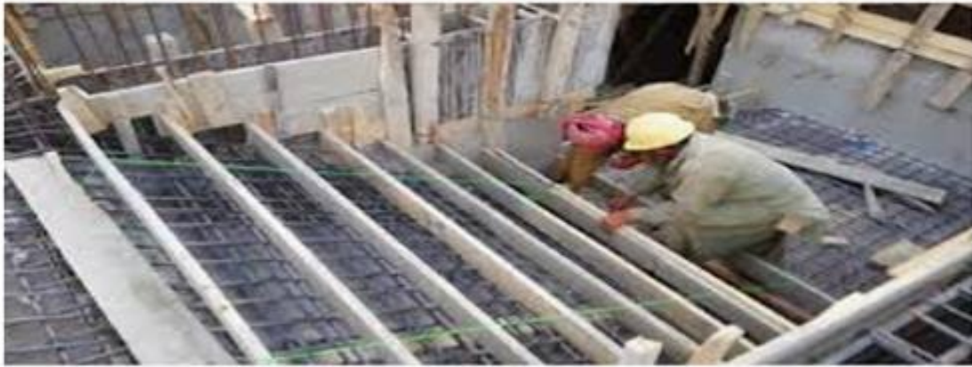
Fig 2.3. Setting out Formwork
