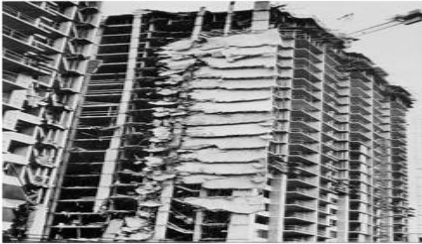
Fig 5.3. Improper Stripping
