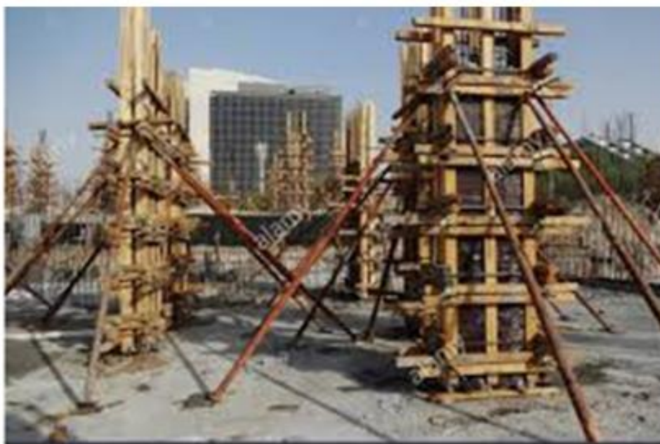
Fig 4.2. | Shuttering
