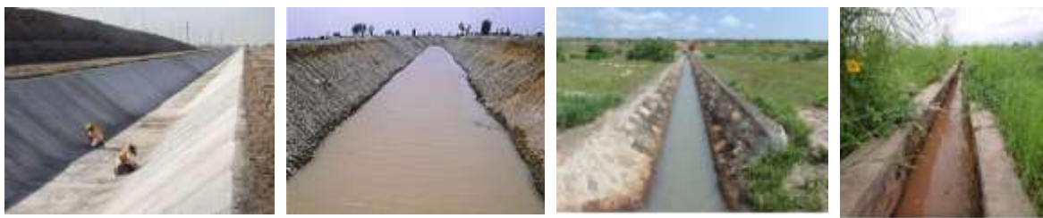
Fig. 1.7: Trapezoidal, rectangular stone paved lined canal for irrigation work
