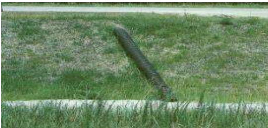
Fig.2.5: Temporary Pipe Slope Drains
