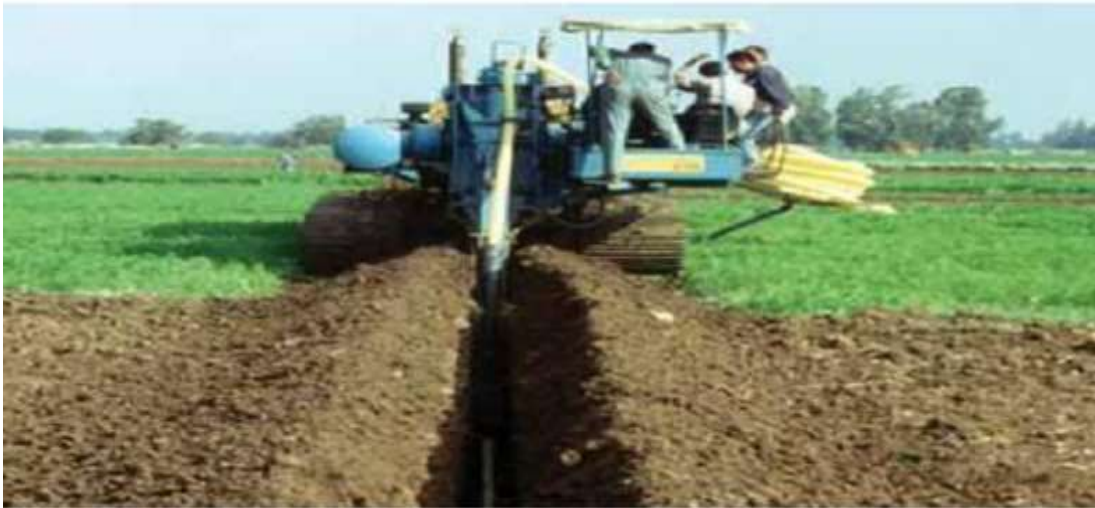
Fig 1.5: Excavating the trench
