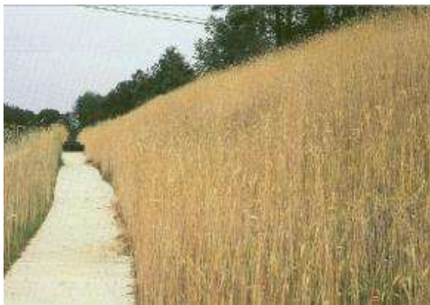
Fig.2.9: Temporary Erosion Control Seeding
