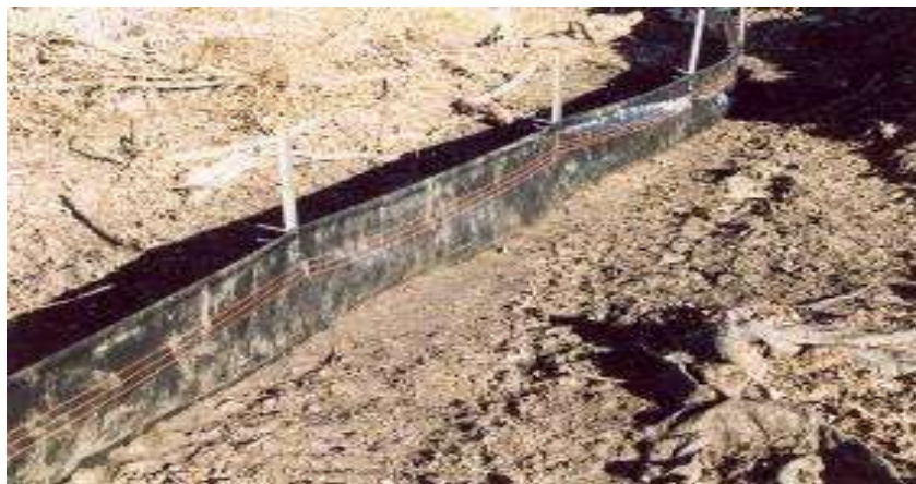
Fig.2.8: Silt fences
