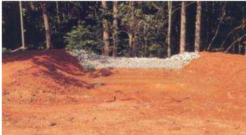
Fig.2.7: Sediment Traps
