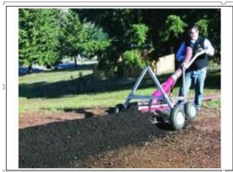
Fig. 2.1: filter berm
