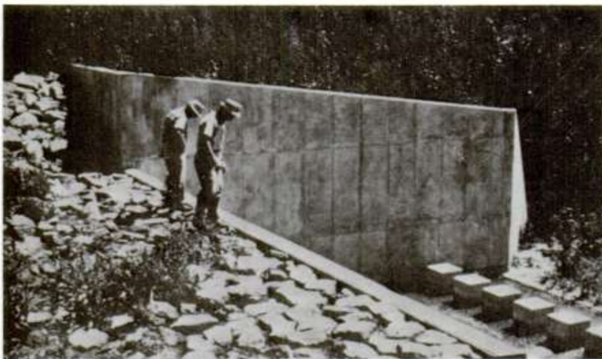
Fig.2.2: Concrete check dam
