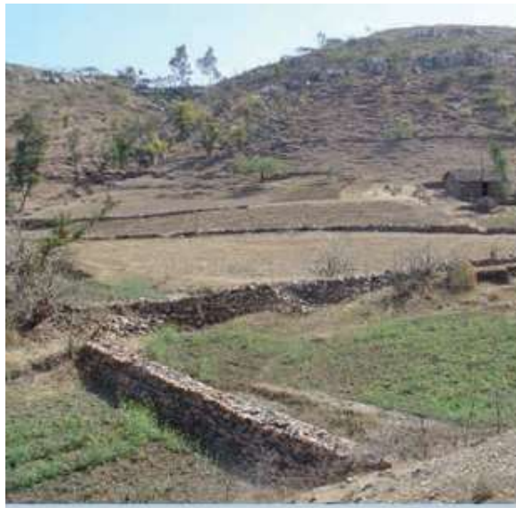
Fig. 4.1. Permeable Rock Dams.
