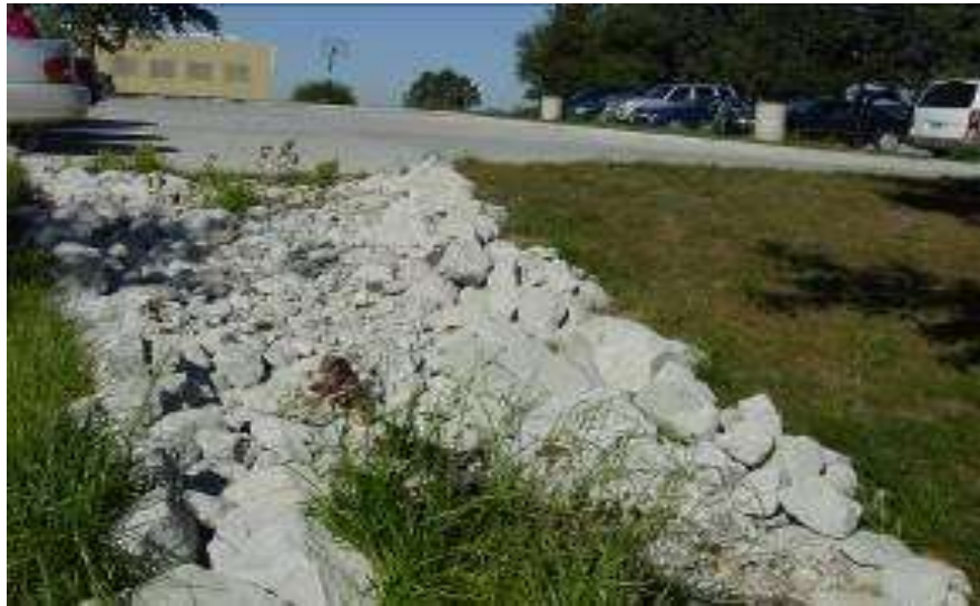
Fig.2.13: Rock chutes and flumes
