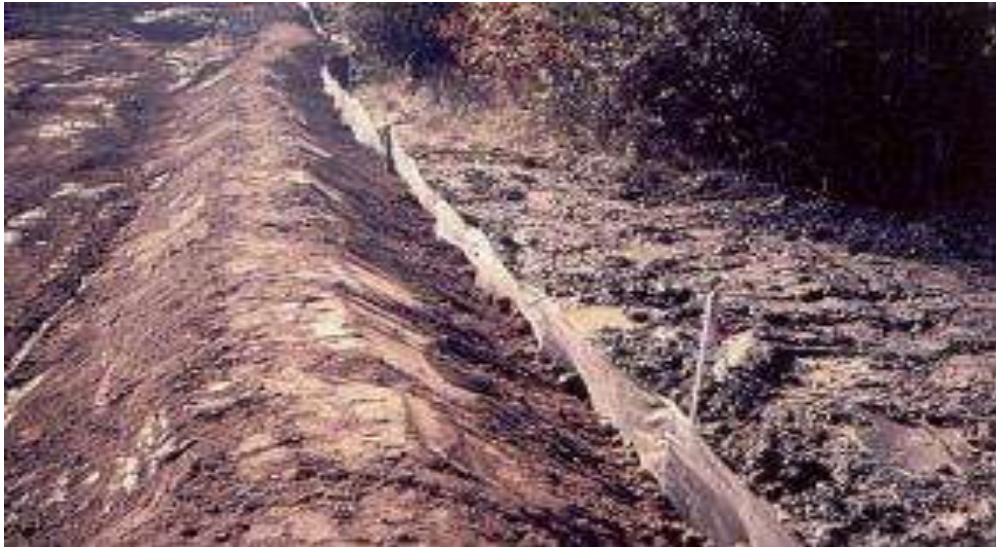
Fig 2. 3: Temporary earth diversion structures
