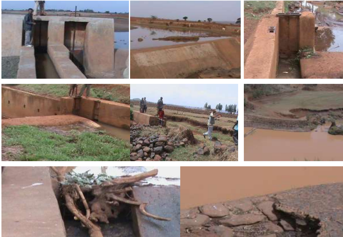
Fig. 2.1: Different problems on diversion weir structures
