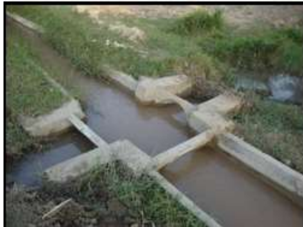
Figure 1.9: Water distribution system in Surface Irrigation
