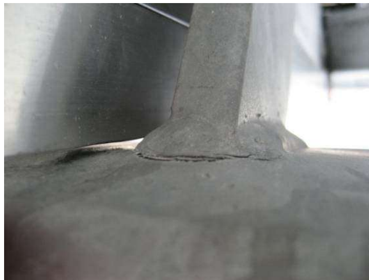
Image 4: Crack damage – fixing system
