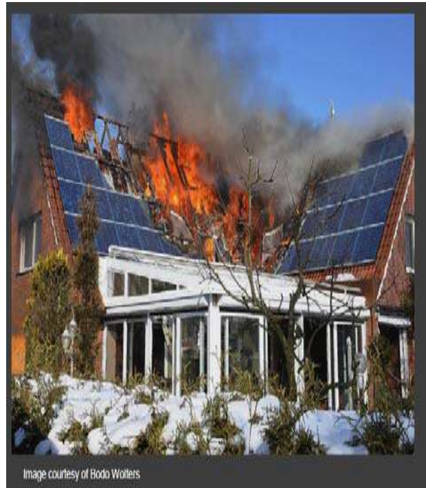
Image 1: Owners should stay away from the PV system during and after a fire and inform the fire brigade about the particular hazards from the PV system.
