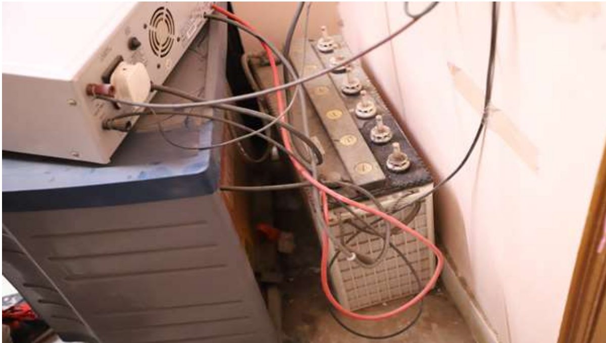
Figure 53: Solar Inverter and Solar Battery Connection
