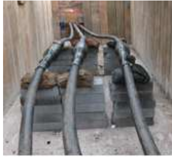
Figure 32: HV cable jointing and laying
