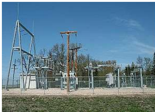
Figure 27: Example of 115 kV to 41.6/12.47 kV 5 MVA 60 Hz substation
