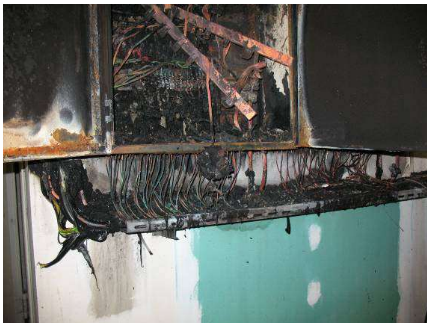
Image 2: Improper wiring method
