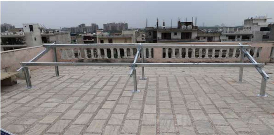
Figure 49 :Roof top Solar Mounting Structure
