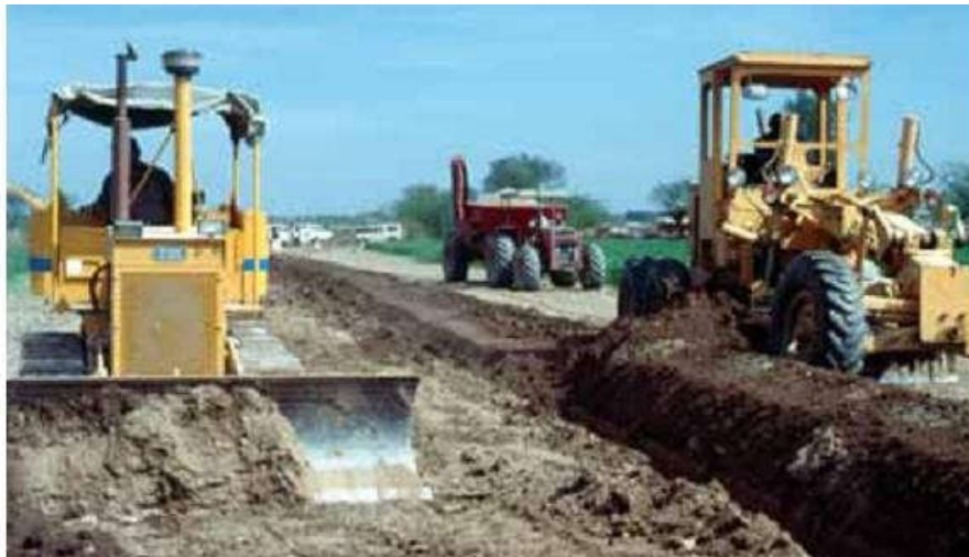
Figure_2.5: Backfilling of the drain: using a dozer and grader
