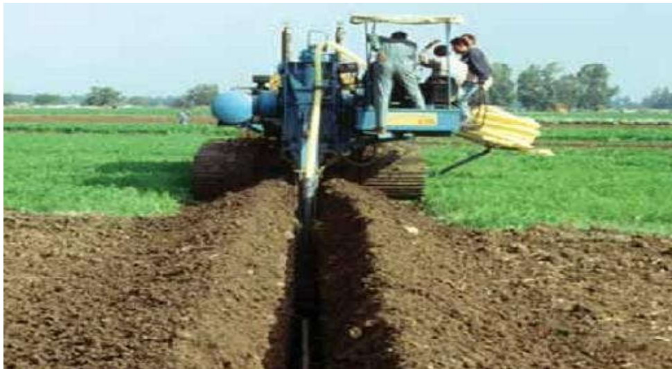
Figure_2.2: Excavating the trench
