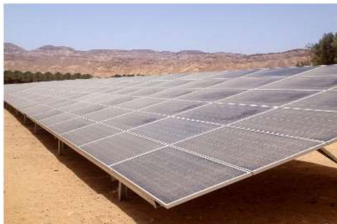
Figure 20: Power plant in Israel, with soiling losses measured > 20\%
