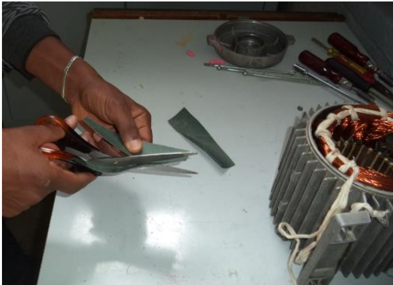
Figure 3.4 insulation preparation
