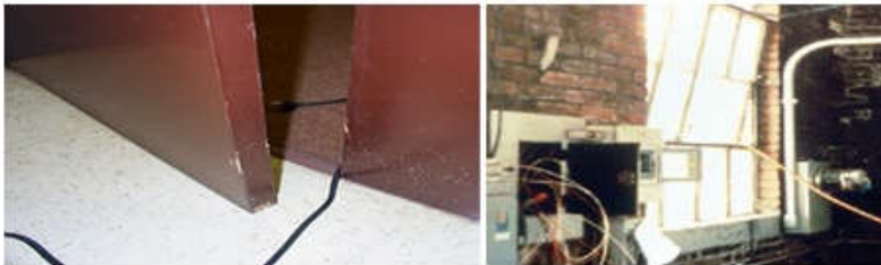
Figure 2. 7damaged Cords
