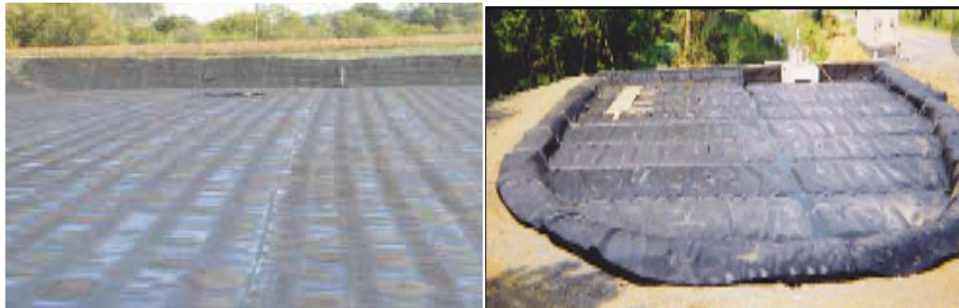
Figure 28: Closed-cell floating cover
