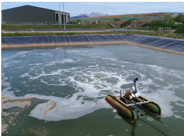
Figure 32-A: Floating aerators for liquid waste aeration
