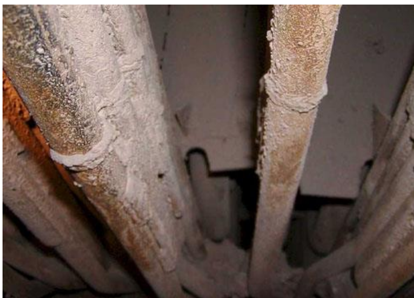
Figure 3.22 Another view of refractory seals that must be replaced. Courtesy:
