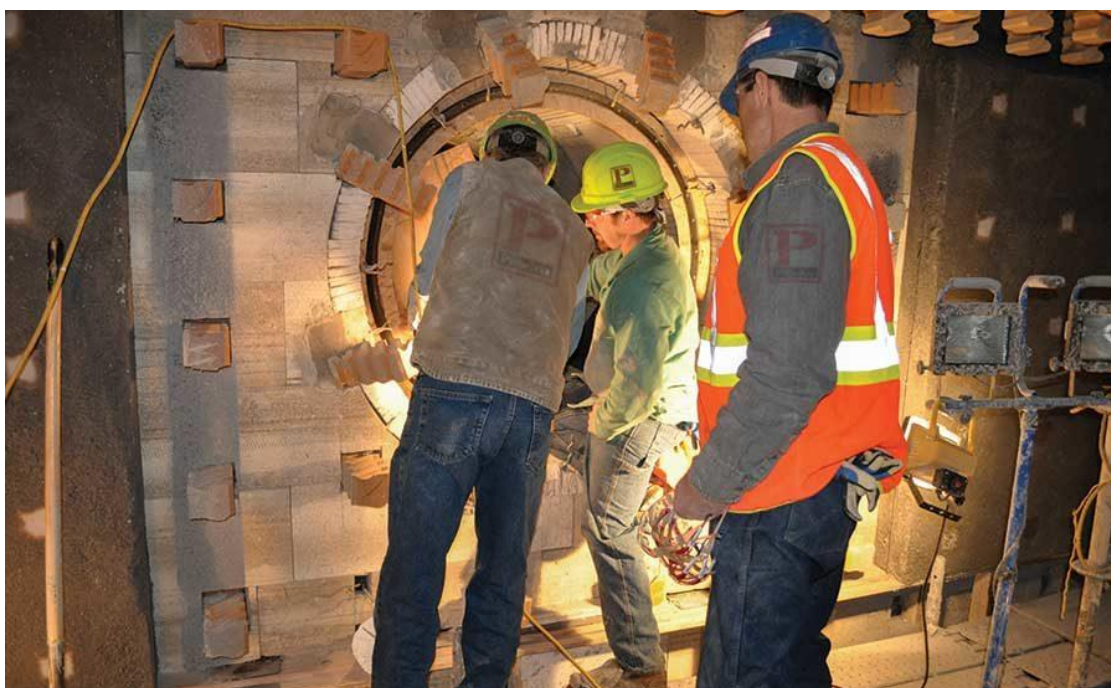
Figure 4.2 refractory lining installation
