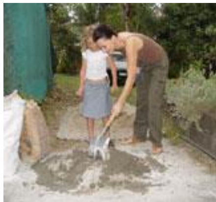
Figure 3 adding more water to refractory concrete
