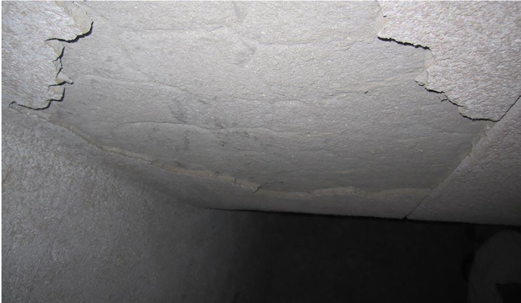
Figure 1.10 Convection Castable/Corbel Damage
