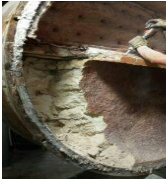
Figure 2.1 manual refractory removing
