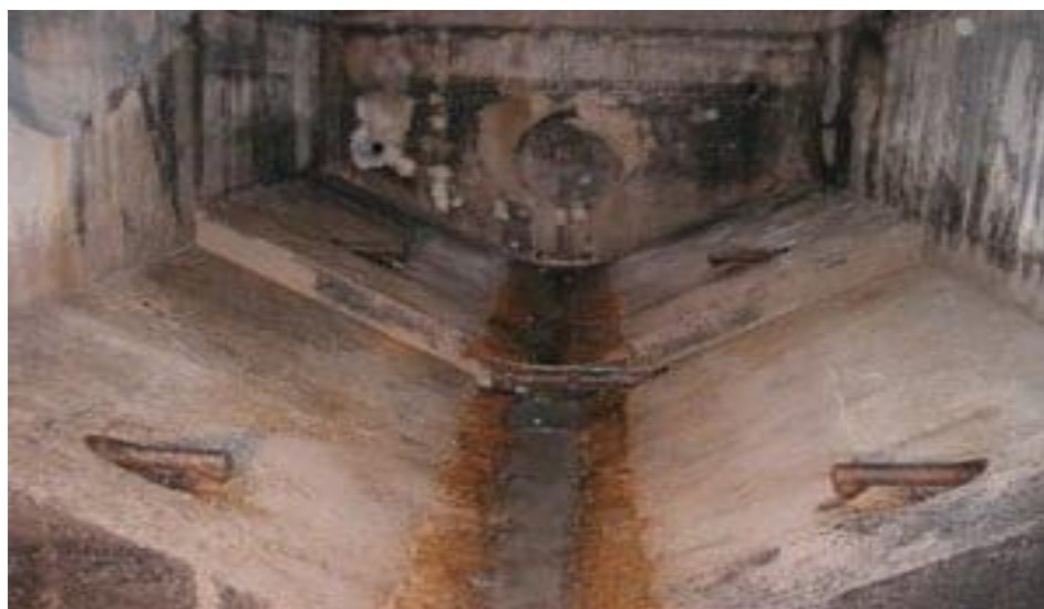
Figure 1.6 Unprotected section. A wet bottom-ash hopper with areas of missing refractory
