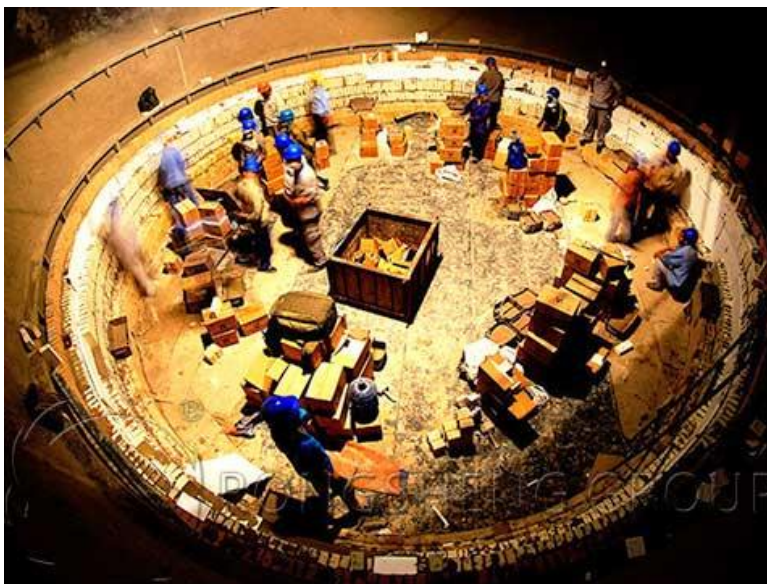
Figure 1.3 Construction Refractory Lining for Blast Furnace
