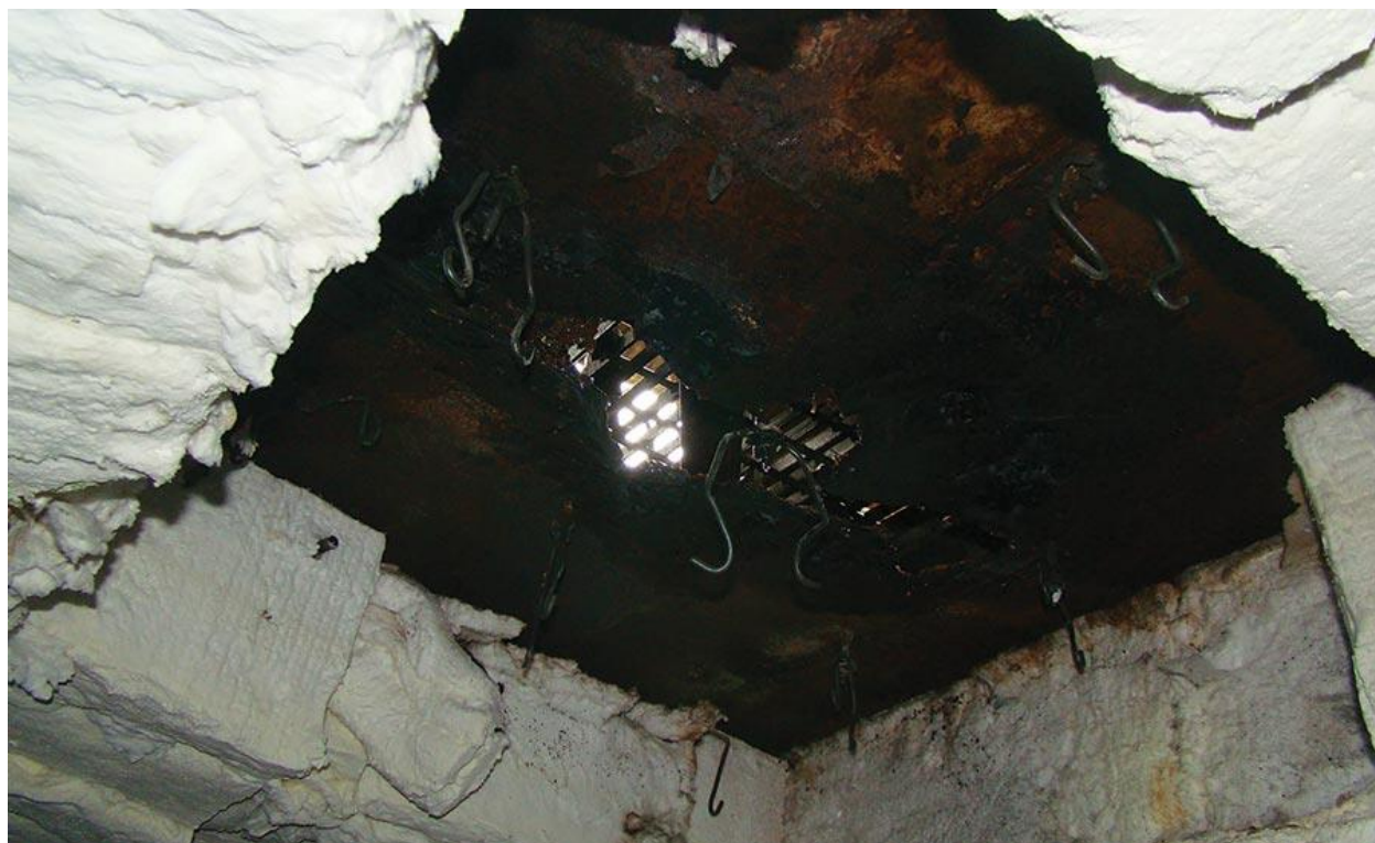
Figure 1.8 Fiber Modules Fallen from the Roof
