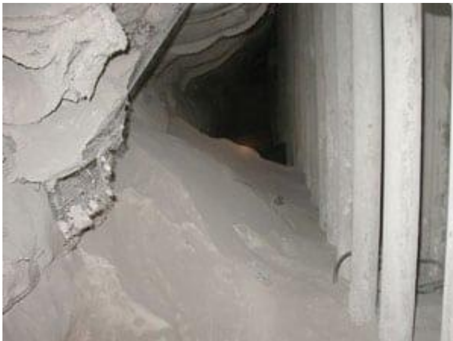
Figure 1.7 Fly ash inside a penthouse between the screen, super heater, and re-heater.
