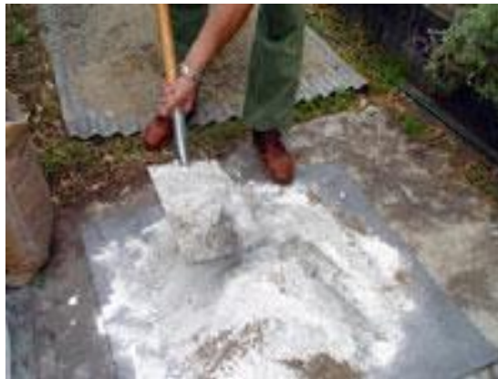
Figure 3.14 Mixing dry refractory concrete ingredients
