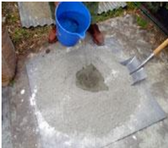
Figure 3.15 Adding water to refractory concrete
