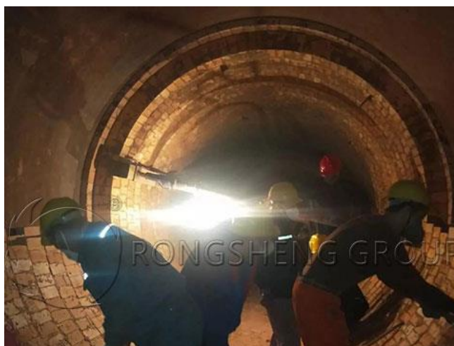
Figure 1.5 Cement Kiln Refractory Lining Construction
