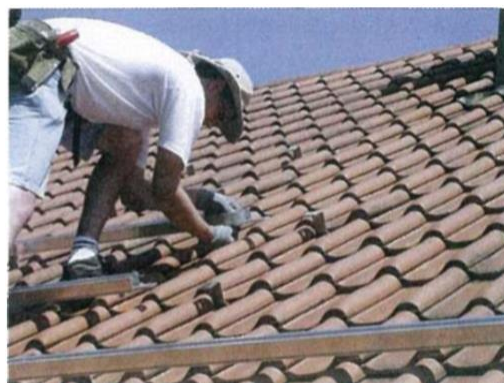
Figure 4 : tile cutting
