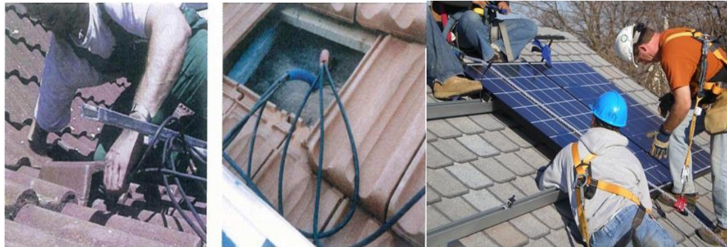
Figure 7 : Running the string cables through the roof
