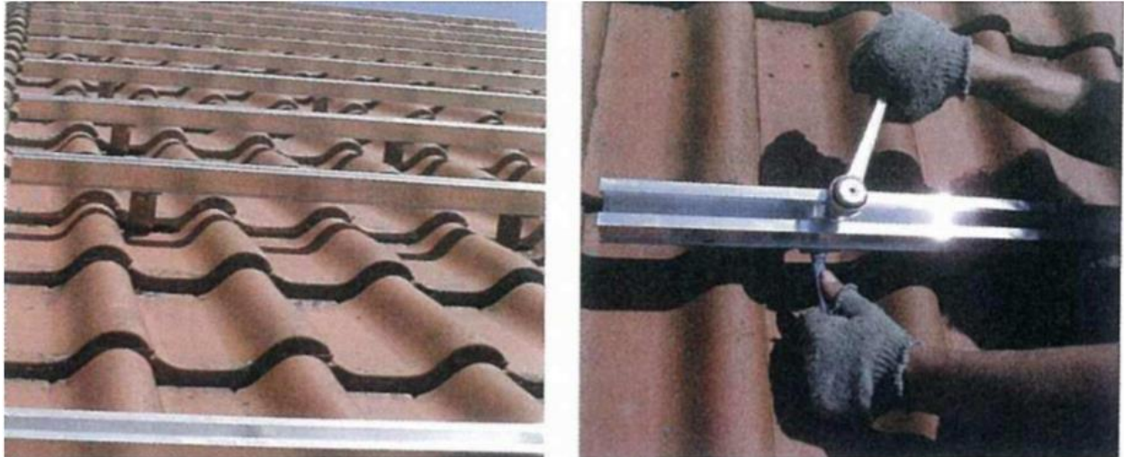
Figure 5 : FIXING RAILS
