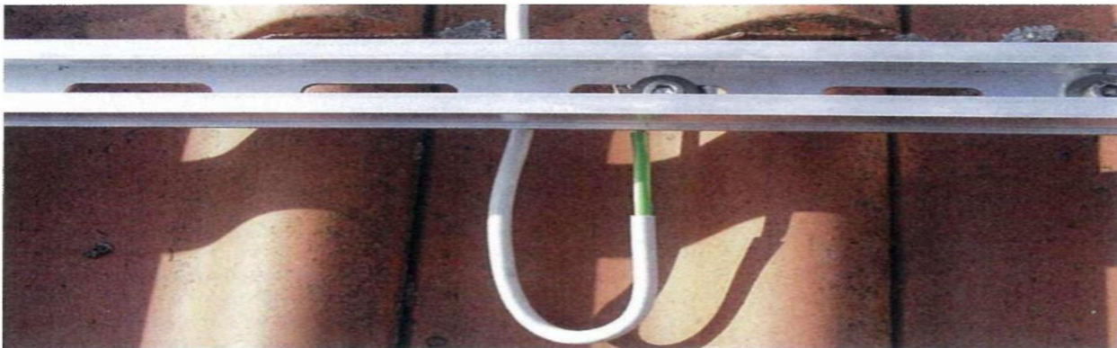
Figure 6 : Earthing/grounding
