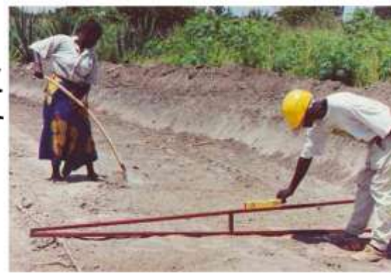
Figure.19.Check camber slope with camber board
