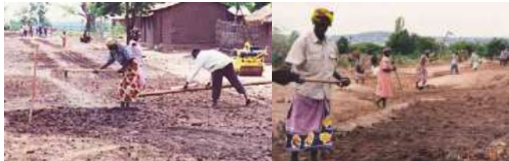
Figure.11. Excavation to level operation
