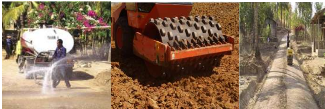
Figure3. Watering and compaction procedure
