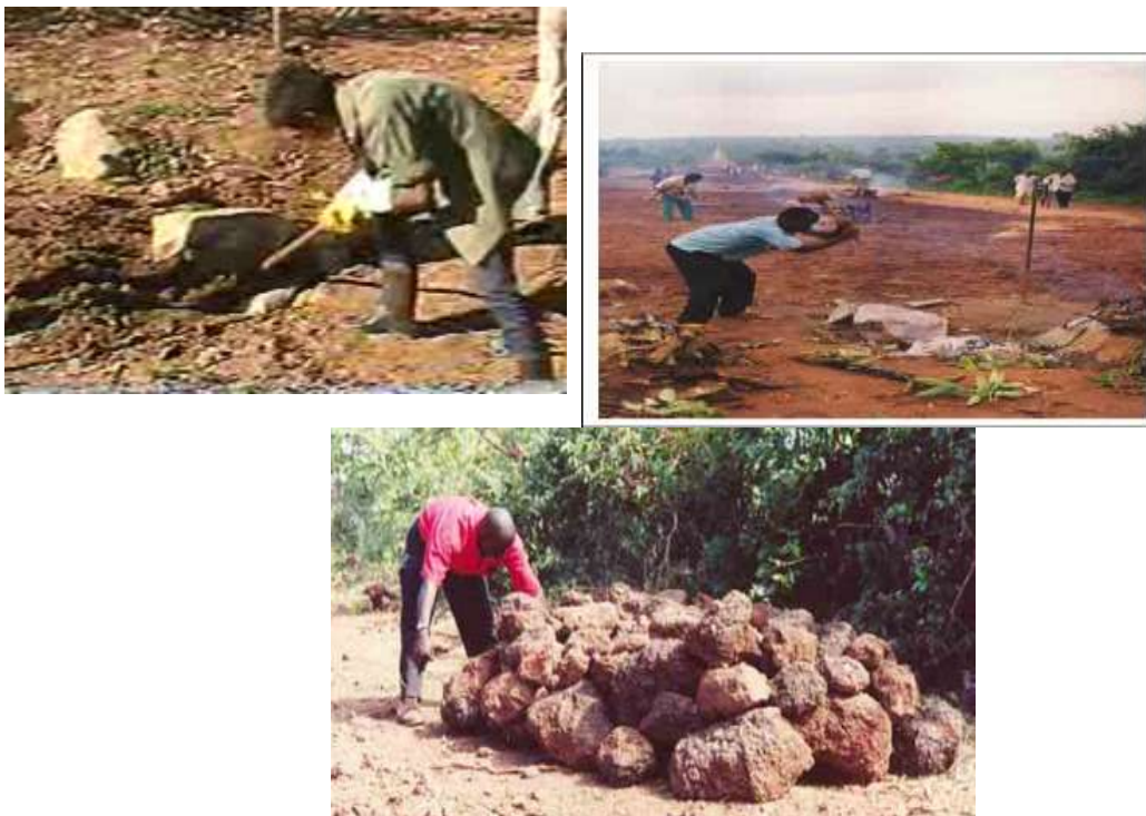
Figure 7. Boulder removal
