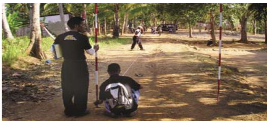
Figure.1 Setting out of road cross section
