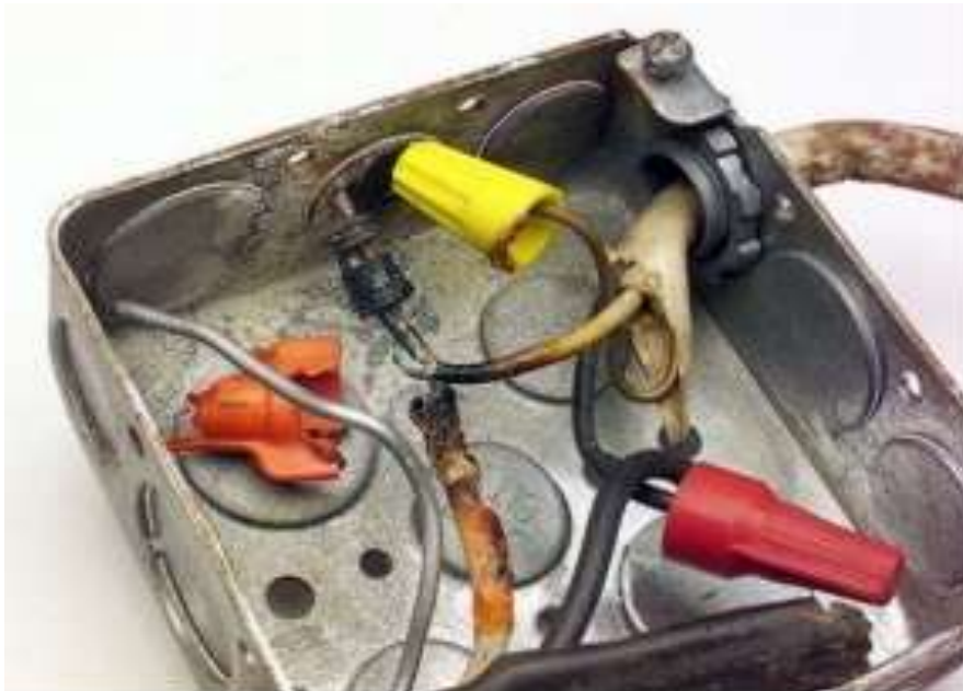
Fig 4.1 heat to burn up the connection wire
