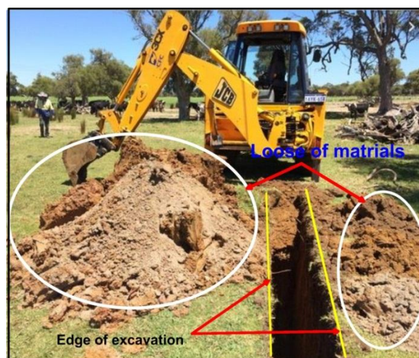
Fig 1.1. Edge of trench with its loose material
