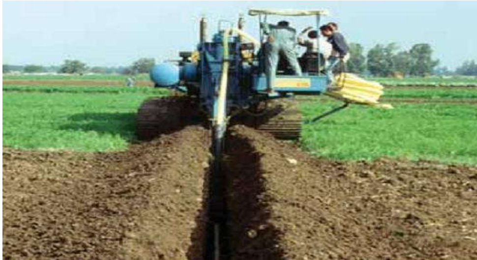
Figure_6: Excavating the trench
