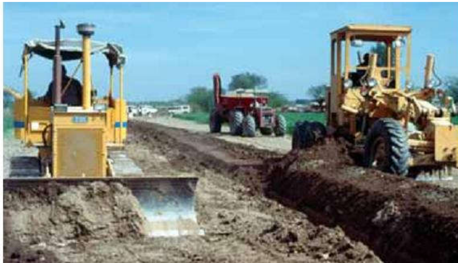
Figure_9: Backfilling of the drain: using a dozer and grader
