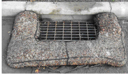
Fig 2.1 Inlet protection
