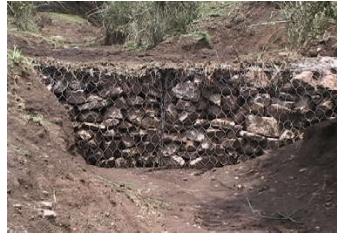
Fig 2.6 gabion check dams
