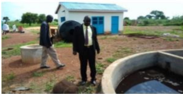
Fig.2..15. Poor separation of liquid and solid wastes from slaughterhouse
