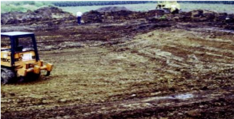
Figure 2.14: The sod and topsoil in a pond construction area can be stockpiled for later use
