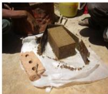
Step 4. Removing block from the mold
