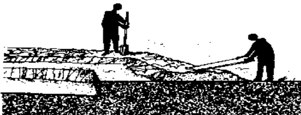
Figure 2.11: Compacting the pond dyke (embankment)
