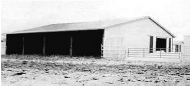
Figure 1b: Open sided, clear span pole shed
