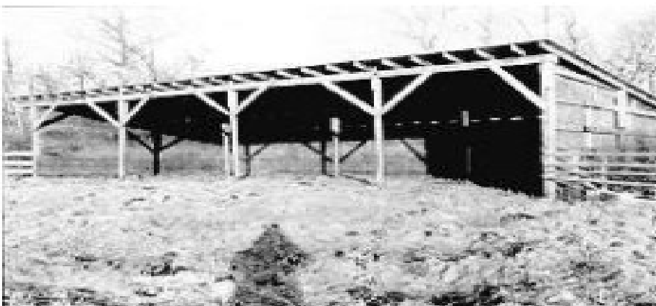
Figure 1a: Open sided, single slope roof shed
