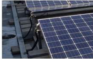
UV protection for exposed cables and max. bending radius
