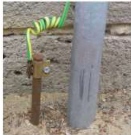
Figure 16: Grounding electrode
