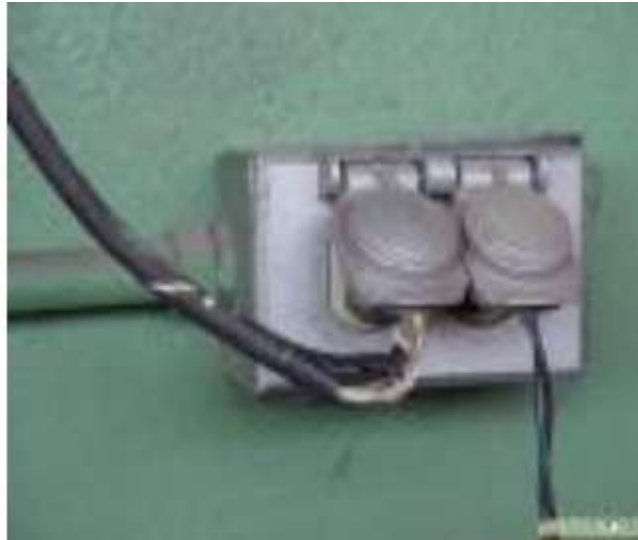
Figure 5: Figure Damaged Insulation and Plug
