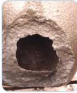
Fig. 4.1. The impact of charge material dropped into the crucible produced this damage
