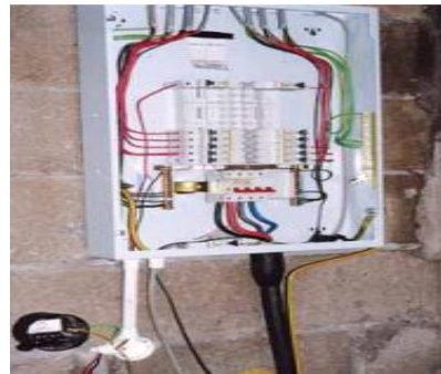
Figure 1.4 Wrong installation of socket out let from distribution board
