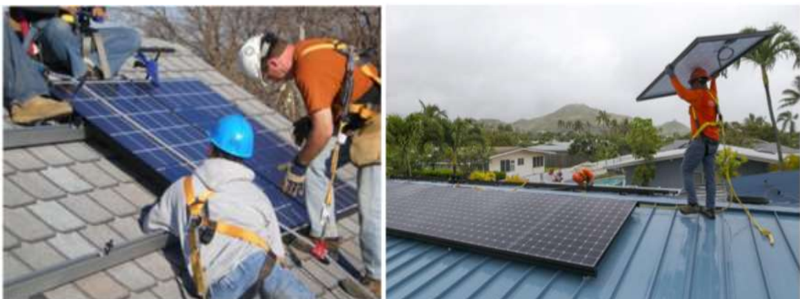
Figure 12: Proper PPE wiring while working on rooftop PV systems (GIZ, 2016)
