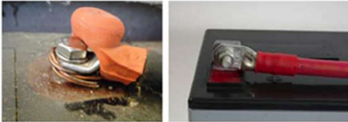
Figure 19: Poor connection (left), good connection (right)
