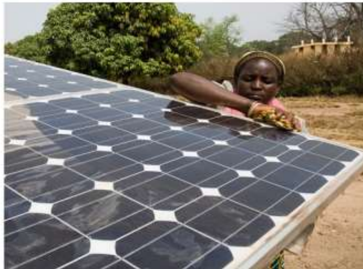
Figure 17: Dusty solar panels being washed
