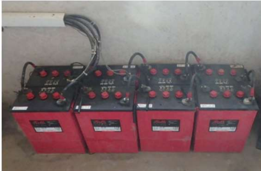
Figure 16: A 48 V battery bank for a mini-grid in Kenya consisting of a string of eight, six-volt batteries arranged in series
