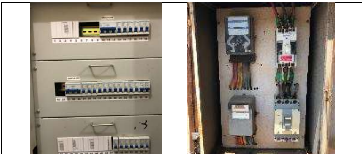
Fig: Pictures from distribution board and meter
