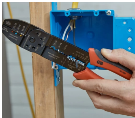
Figure 11: Prepare the Bare Ends of the Wires
