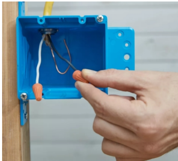
Figure 12: Place Wire Nuts on the Wires
