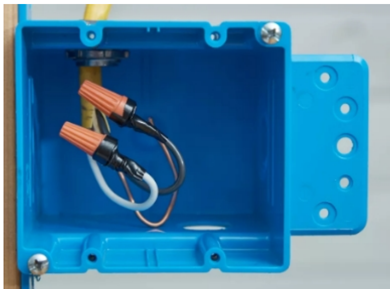
Figure 13: Push the Wires into the Box
