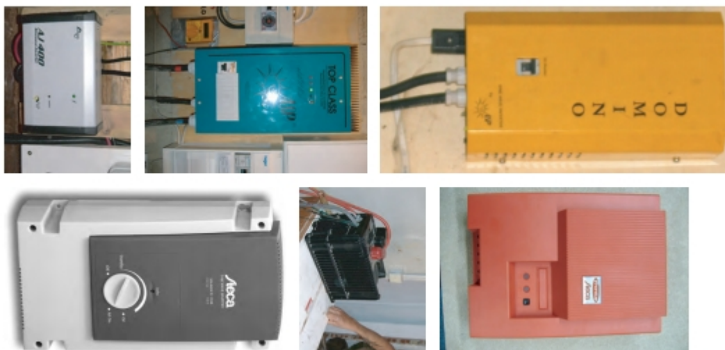
Figure 21: Common sine wave inverters used in PV systems: Solon ASP Domino, 600W at 12V, 1000W at 24V (top left); Steca Fronius Solaris IP, 500W, version with integrated solar charge controller available (top right); Solon ASP Top Class, 1000W (middle left); Outback inverter with integrated
