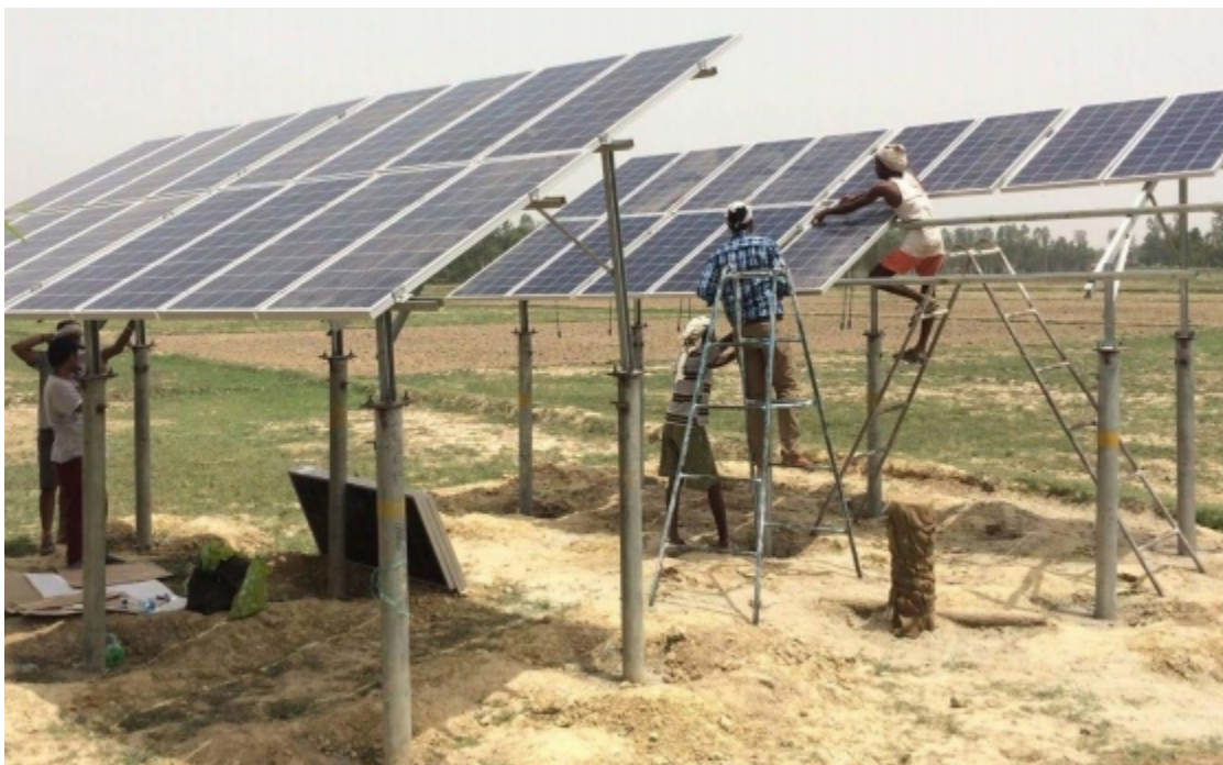
Figure 35: Solar panel installation.
