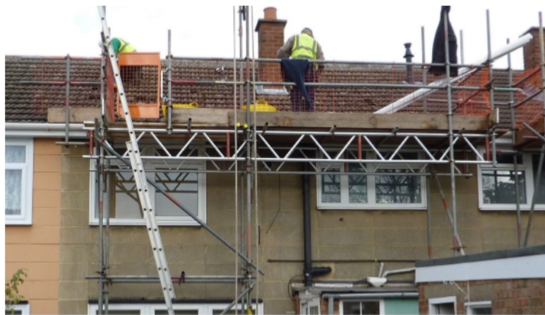
Figure 14: Acceptable edge protection
