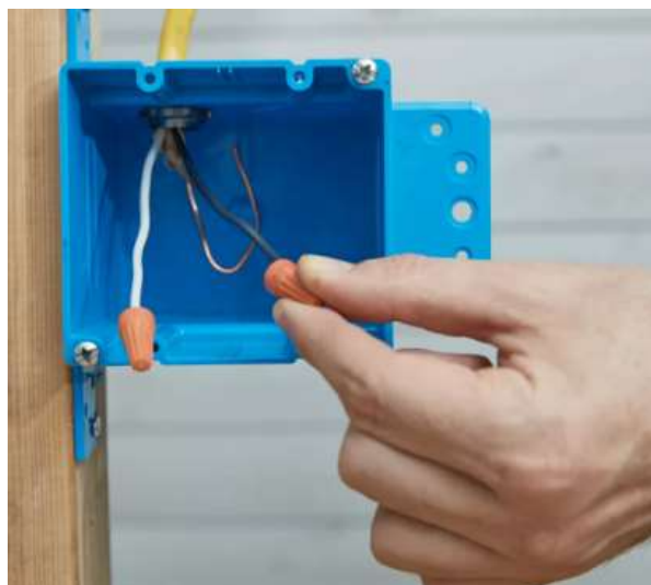
Figure : Place Wire Nuts on the Wires
