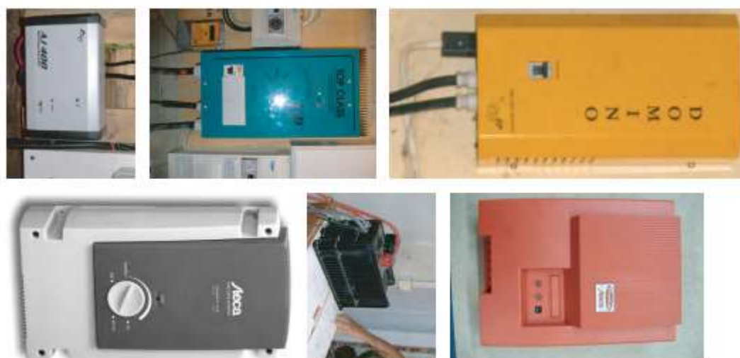
Figure : Common sine wave inverters used in PV systems: Solon ASP Domino, 600W at 12V, 1000W at 24V (top left); Steca Fronius Solaris IP, 500W, version with integrated solar charge controller available (top right); Solon ASP Top Class, 1000W (middle left); Outback inverter with integrated battery charger for charging batteries from generator, 2000W (middle right);
