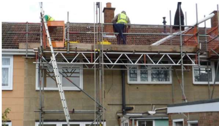
Figure : Acceptable edge protection
