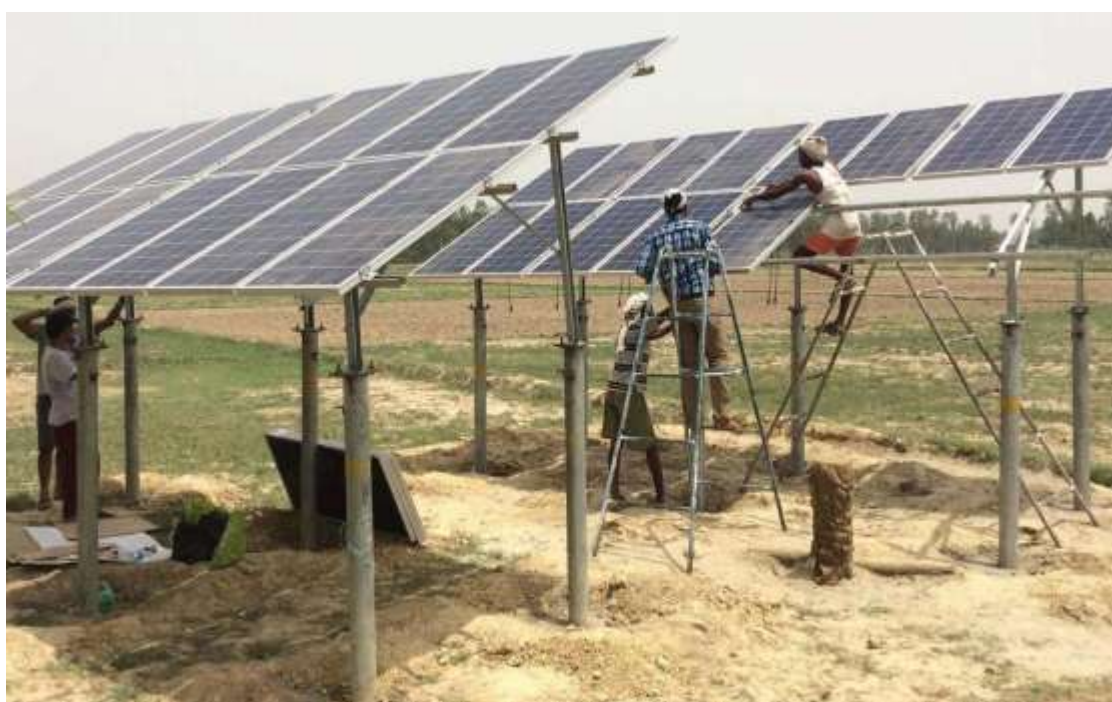
Figure : Solar panel installation.
