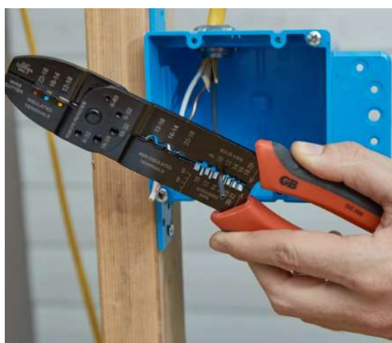
Figure : Prepare the Bare Ends of the Wires
