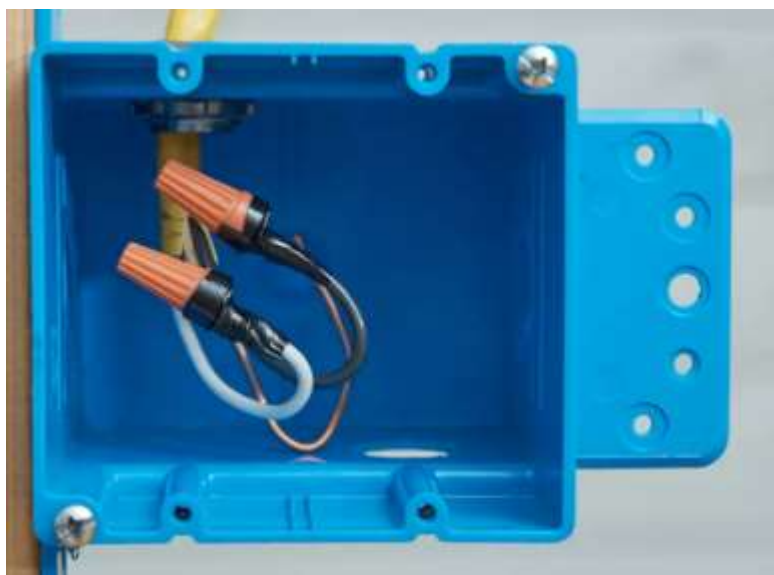
Figure : Push the Wires into the Box
