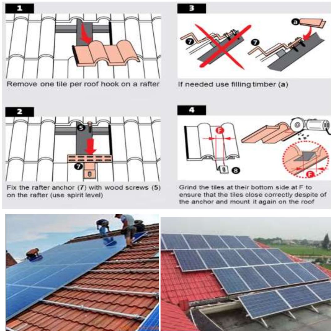
Figure 18: Installing roof hooks instructions ( https://www.solarmango.com/scp/mounting-structure-supporting-the-solar-panels-on-the-ground/ )
