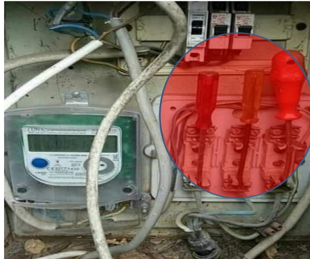
Figure 70: Dangerous fuse 'replacement'
