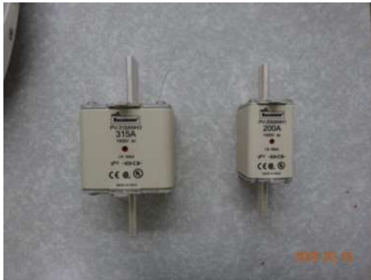
Figure 71: Battery DC-rated fuses
