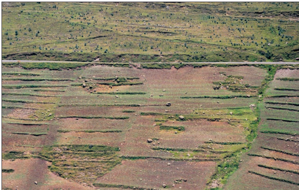
Photo 10.1: Selective removal of SWC structures – a first step to a new SWC system
