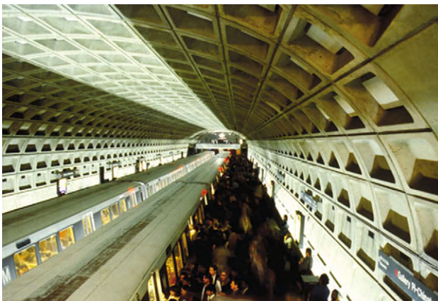
FIGURE 8.1 Precast lining in a metro tunnel. (source: http://www.railwayage.com/sept01/washmetro.html )
