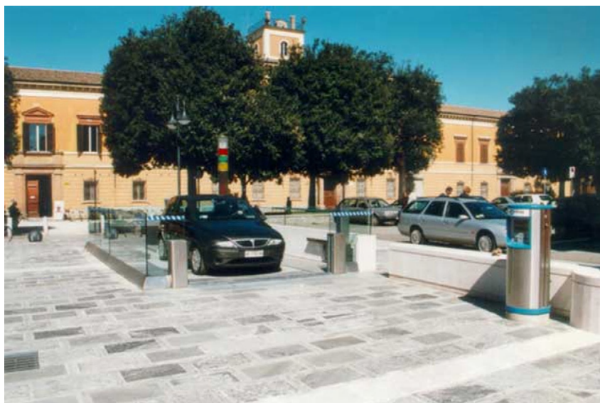
FIGURE 7.5 Trevipark system with direct loading bay for 84-car parking capacity underground. (source: www.trevipark.co.uk )
