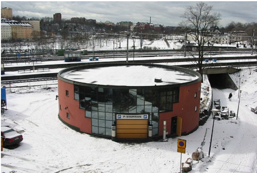
FIGURE 7.3 Trevipark system with 47 car capacity; 23 aboveground and 24 underground. (source: www.trevipark.co.uk )
