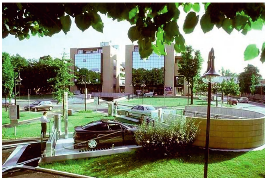
FIGURE 7.4 Trevipark system with indirect loading bay for 72 cars underground. (source: www.trevipark.co.uk )
