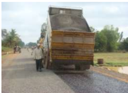
Stone chipping (aggregate) applied uniformly after bitumen spray
