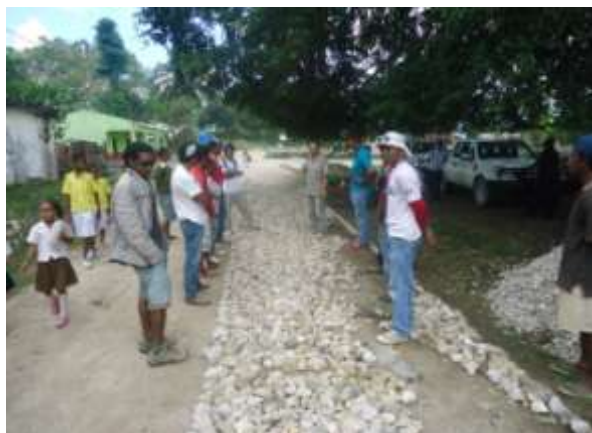
Aggregate layers – base, intermediate and surface
