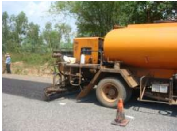
Even application all spray nozzles
