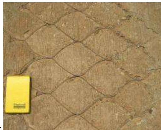
Geo-cells 2 years after construction
