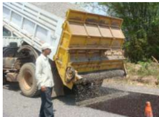
Mechanical spreader and speed of truck governs application
