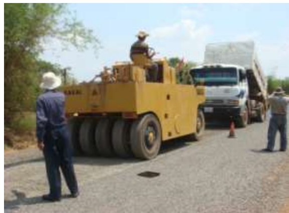
Roll with pneumatic tyre or smooth wheel tandem roller
