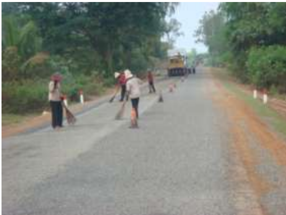
Sweep stone chippings or broadcast additional for even coverage
