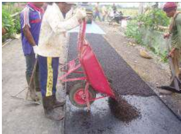
Placing material mixed in mixer, and spreading
