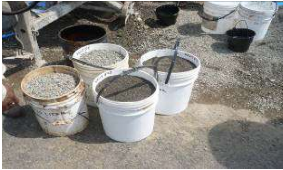
Materials batched for mixing and concrete mixing
