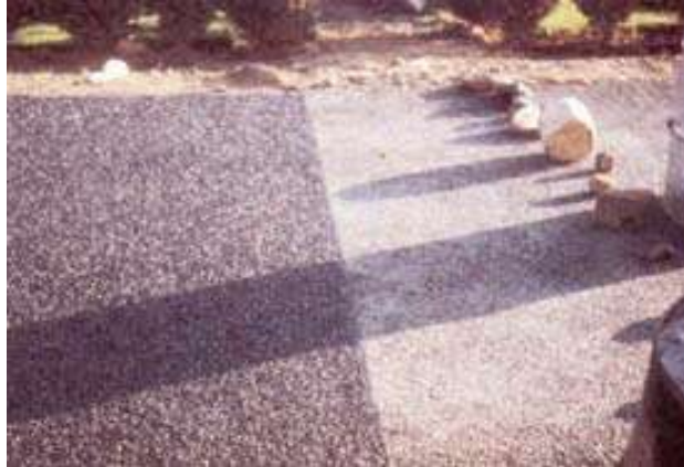
Neat construction joint due to use of reinforced paper
