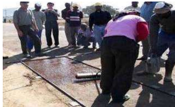
Guiderrails placed, tack coat applied
