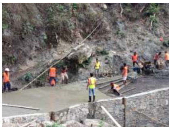
Steel mesh reinforced concrete pavement construction in Timor-Leste
