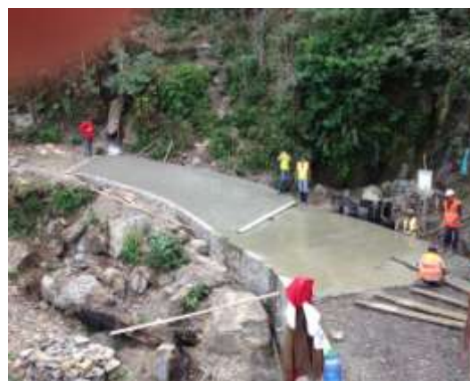
Steel mesh reinforced concrete pavement construction in Timor-Leste
