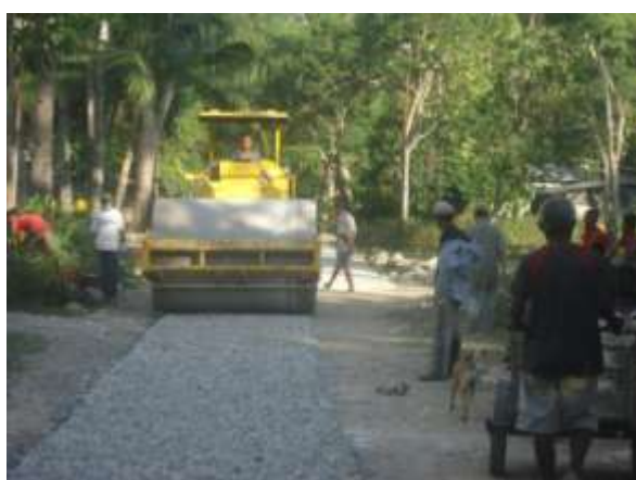
Rolling intermediate layer; applying penetration coat for surface layer
