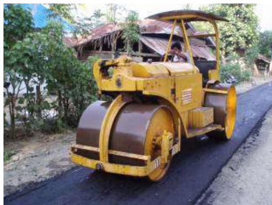
Spreading and rolling Latasir mix
