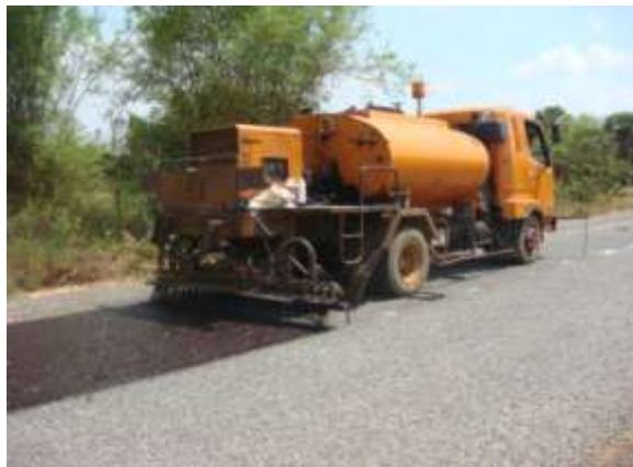
Spray run marked with guide for driver
