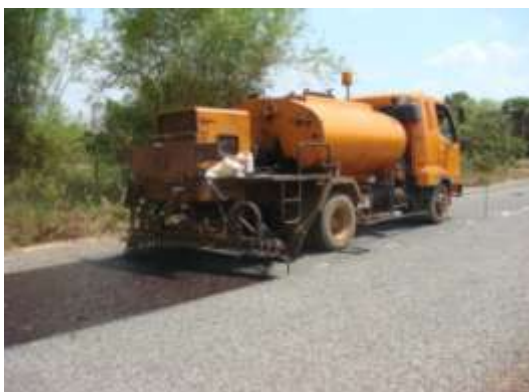
Even application from all spray nozzles
