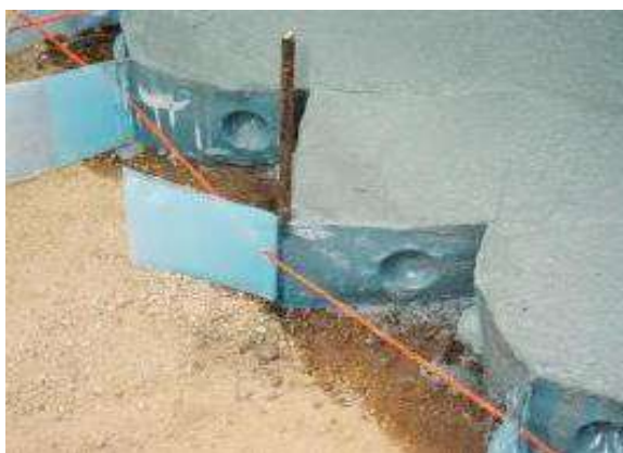
Geo-cells during Construction
