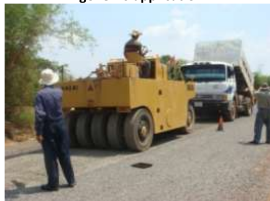
Mechanical spreader and speed of truck governs application
