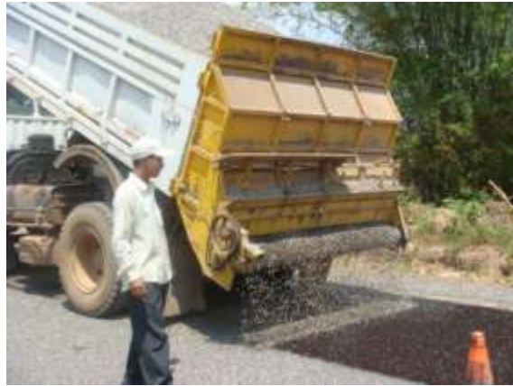
Application of aggregate
