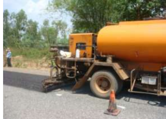
Spray run marked with guide for driver
