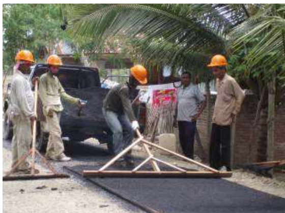
Spreading and rolling Latasir mix
