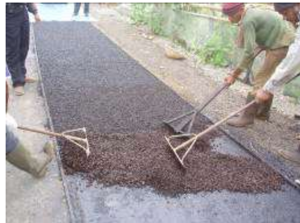
Placing material mixed in mixer, and spreading
