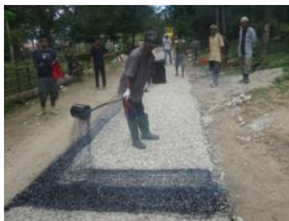
Rolling intermediate layer; applying penetration coat for surface layer
