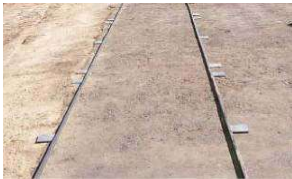
Guiderrails placed, tack coat applied
