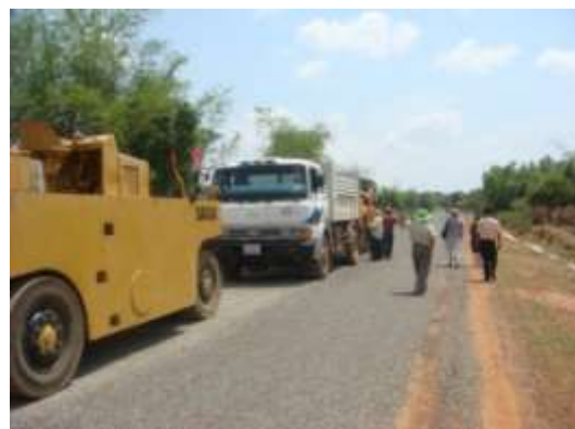
Bitumen run about to start with placement of stone chipping and rolling immediately following application of bitumen binder
