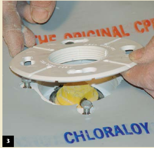
3 Place the retaining ring.
