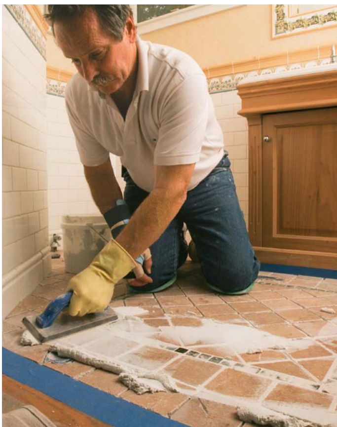
Scoop, spread, and scrape the grout across the floor.
