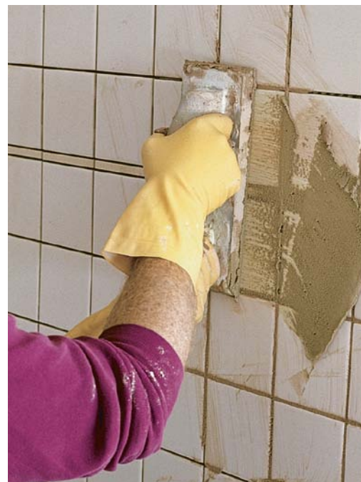
Pack the grout. Hold the trowel at a slight angle and spread grout over a small section. Work grout into the joints until they are full.
