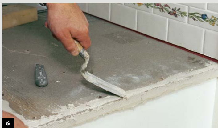
6 Finish edges with thinset. Fiberglass mesh tape and a thin layer of thinset adhesive finish the edges. This substrate is now ready for tile.
