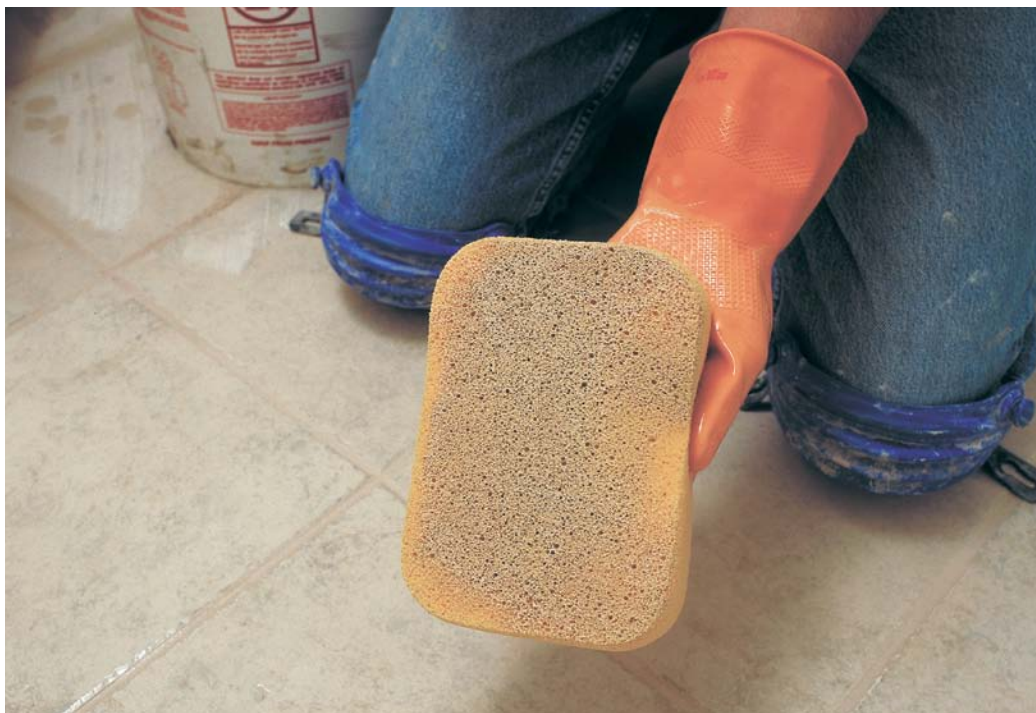
This sponge needs a dunk. After a single light pass across the floor, this sponge has picked up plenty of excess grout. The author flips the sponge over, makes another light pass and then rinses out the sponge.
