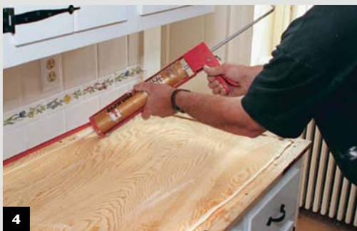
4 Bond the cement board to the counter. A bead of construction adhesive may be used to bond the cement board to the rough top.
