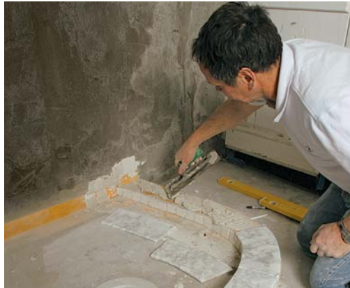
Waterproofed and pitched for drainage. The author uses a waterproof membrane and slightly pitches the marble cap to achieve proper drainage.
