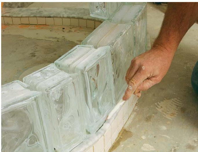
Establish the layout. The glass blocks are first laid dry and then traced with a pencil.
