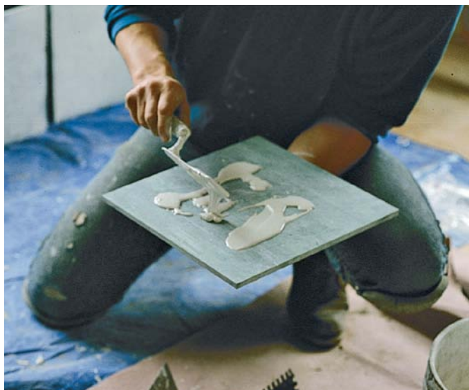
Epoxy seals the backs of the green-marble tiles. Green marble reacts badly to water-based adhesives, so the backs of the tiles are sealed with nonporous epoxy. A trowel spreads the thick and gooey epoxy.
