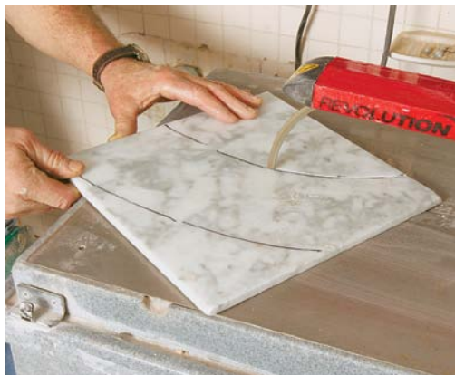
Cut the curves. The author uses a Gemini Revolution tile saw to cut the pieces for the top of the curb.
