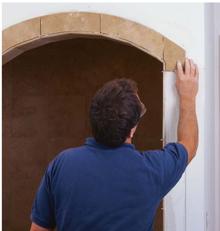
The arch goes up. Once the tiles are shaped and smoothed, they are installed on the wall, leaving the proper spacing for an attractive grout joint.
