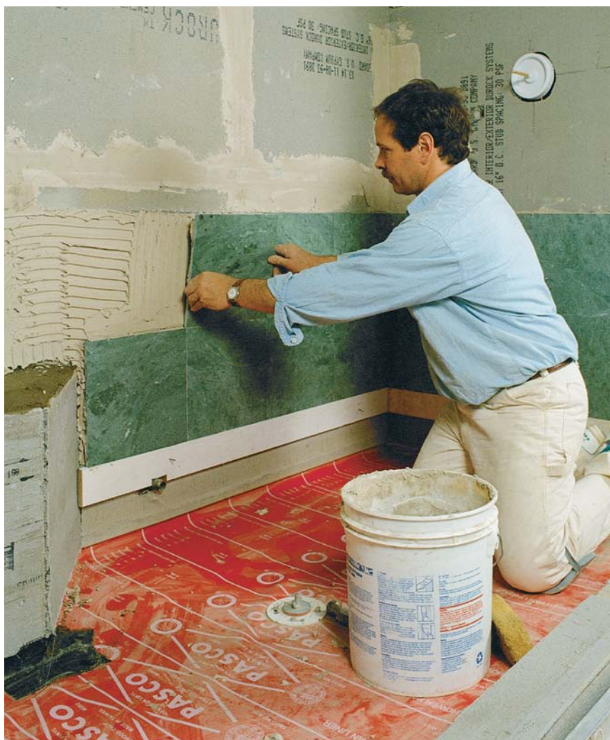
A ledger board keeps the starter course level. A length of 1x is leveled and tacked to the wall to provide support and alignment for the starting course of tile.
