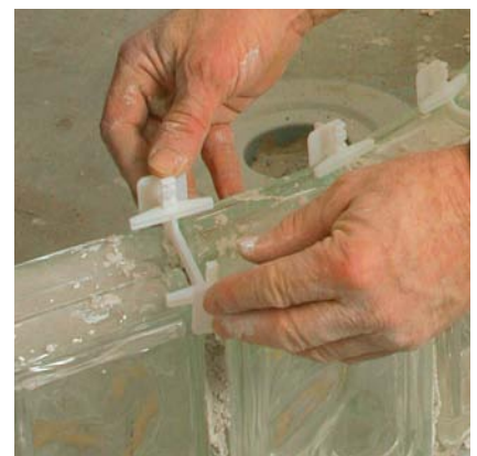
Be aware. Both the straight run glass-block spacers (left) and those for curves (right) look very similar.
