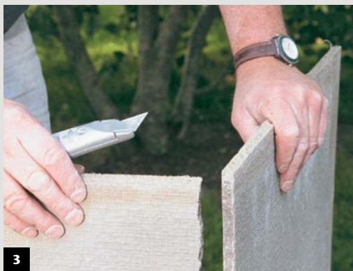
3 The board should break cleanly. Once fibers on the back of the board have been severed, the sheet should break cleanly along the score line.
