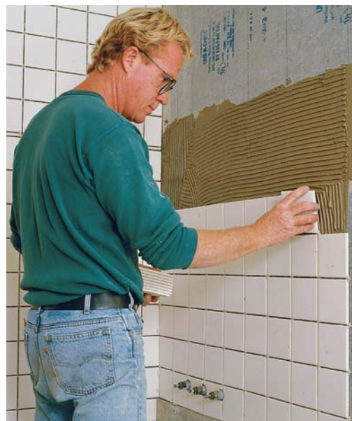
Setting the tiles. With the bottom of the tile resting on spacer blocks, the author tilts each tile onto the mortar and then presses it home.
