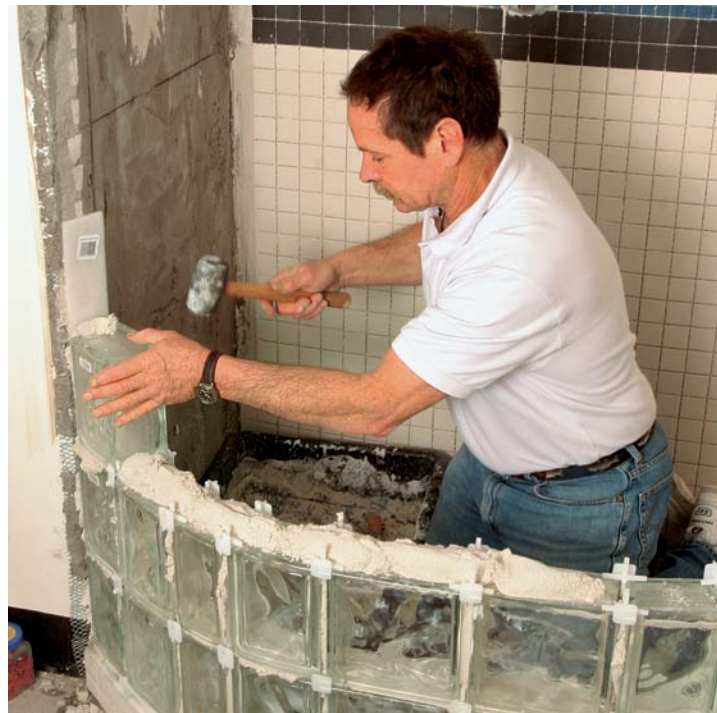
Lock it up. Glass-block spacers lock the blocks in place and keep the grout joint consistent.
