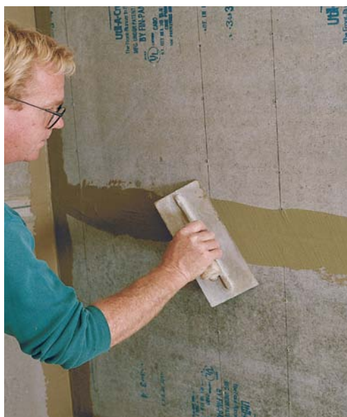
Fill tape with thinset mortar. Use a trowel to spread thinset mortar over taped joints, forcing the mortar into the fabric of the mesh.
