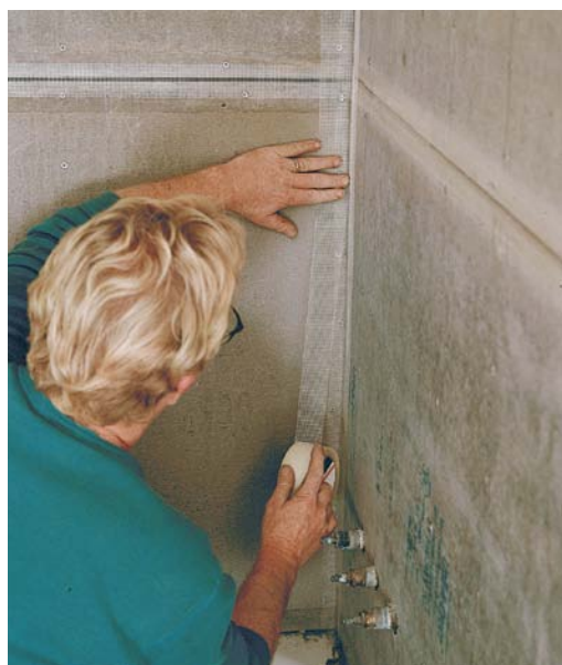
Tape the joints. Press self-adhering, fiberglass-mesh tape over the joints, applying three overlapping strips at inside corners.
