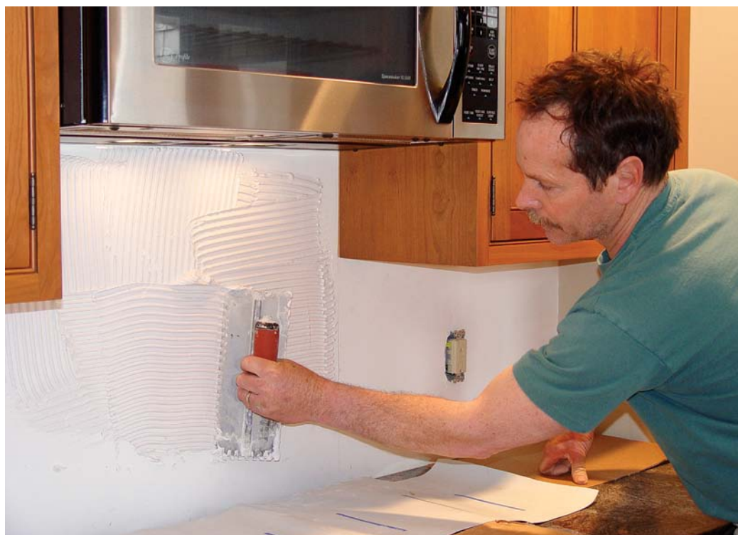
Trowel on the mastic. White mastic is the adhesive of choice for this project because a darker color might show through the light-colored tile. The entire backsplash is spread before any tile is set.
