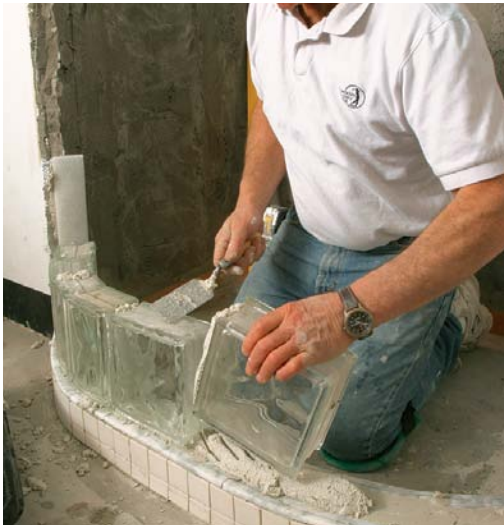
The curb is coated with thinset, then the blocks are set in a thick bed of glass-block mortar.
