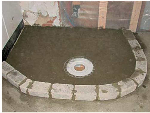
A curved foundation. Landscape blocks are used to create a curved foundation.
