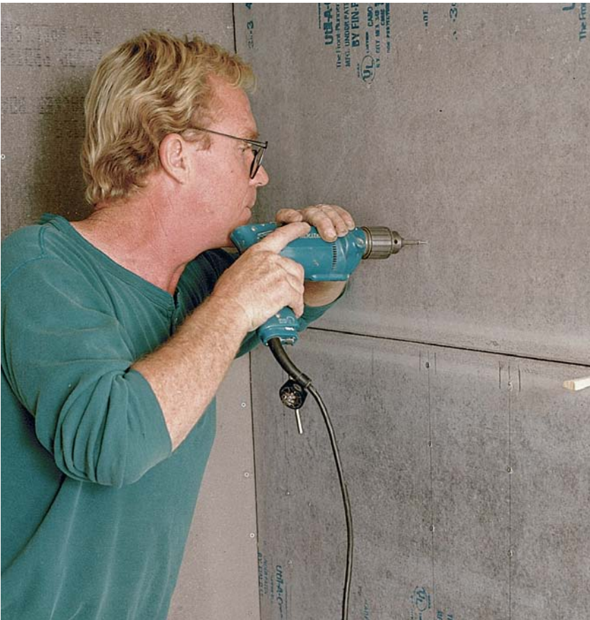
Anchor the backerboard. You can use nails to affix backerboard to the studs, but the board can be damaged during installation. Corrosion-proof screws are a better choice.
