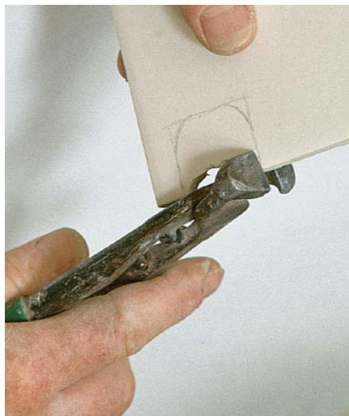
Nibble the notches. Use a biter to notch tiles around plumbing, working in from the corners of the notch to prevent unwanted breakage.
