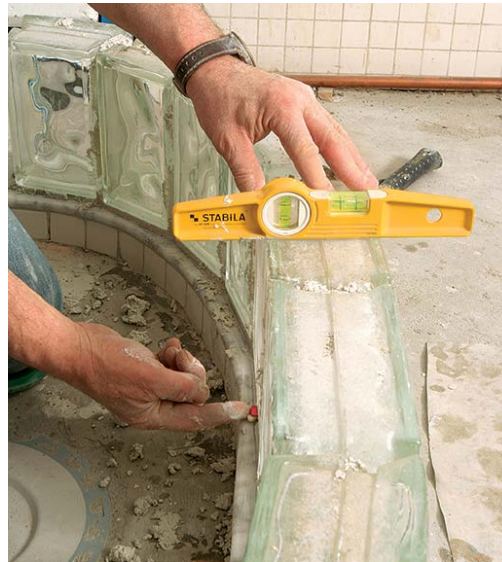
Keep the first course sturdy and level. This first course is crucial, and each block is checked for level.
