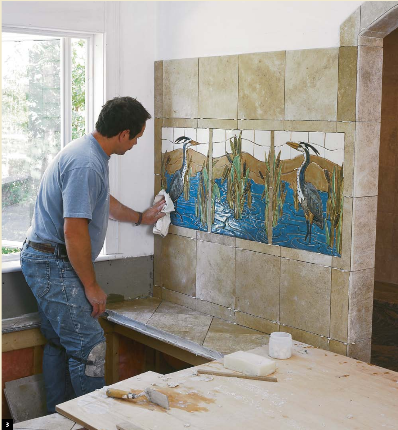
Assembling a ceramic jigsaw puzzle. With the help of a paper map provided by the artist, the installer lays out the ceramic-tile mural carefully on a sheet of plywood (photo 1). After it is laid out, the mural is assembled from its lower corner; the installer works up and over until each section is completed (photo 2). When all the sections are set in place and framed with limestone, a final rinse and wipe down removes excess mortar from the hand-painted ceramic surface (photo 3).
