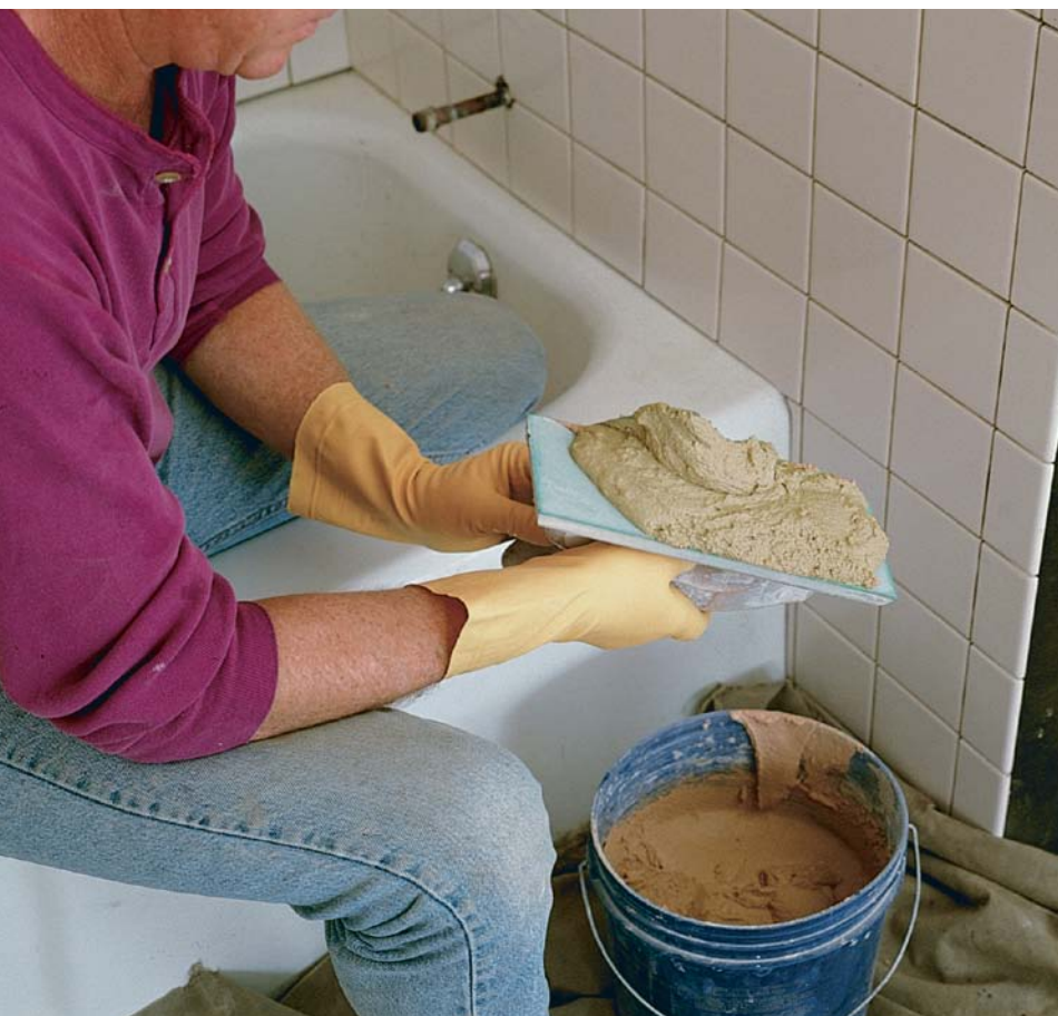
Ready for grout. Load freshly mixed grout onto the rubber face of a grout trowel.
