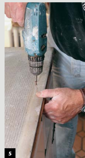
5 Screws hold the cement board down. Galvanized drywall screws 8 in. o.c. keep the cement board in place while the adhesive sets up.
