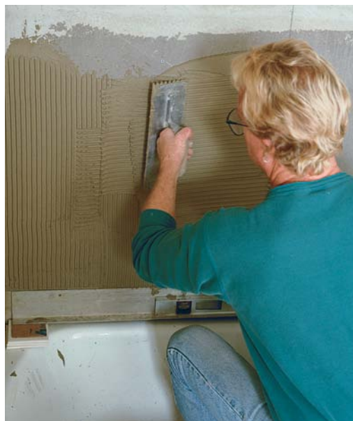
Spreading mortar. Use the straight edge of the notched trowel to spread thinset mortar. Use the notched edge to comb uniform ridges.
