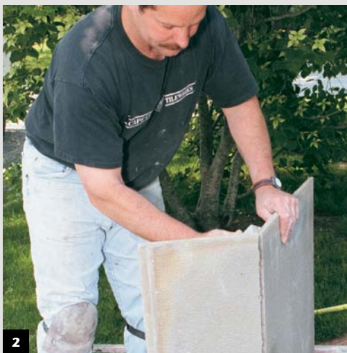
Score the back, too. After snapping the cement board along the score line, Meehan cuts through the back of the sheet, like working with drywall.
