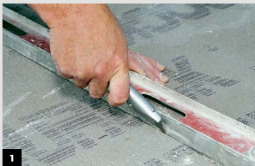
1 Score cement board with a knife. Tilesetter Tom Meehan uses a utility knife and a straightedge to score a piece of Durock cement board.
