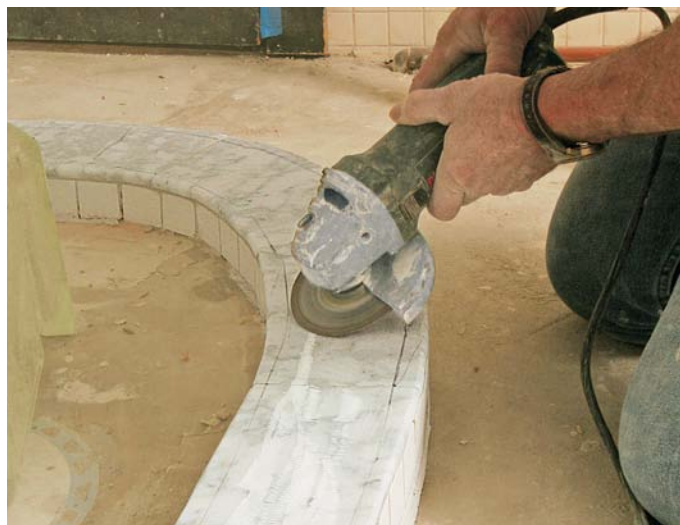
Prep the curb to hold the blocks. The marble cap is scarified in preparation for the thinset.
