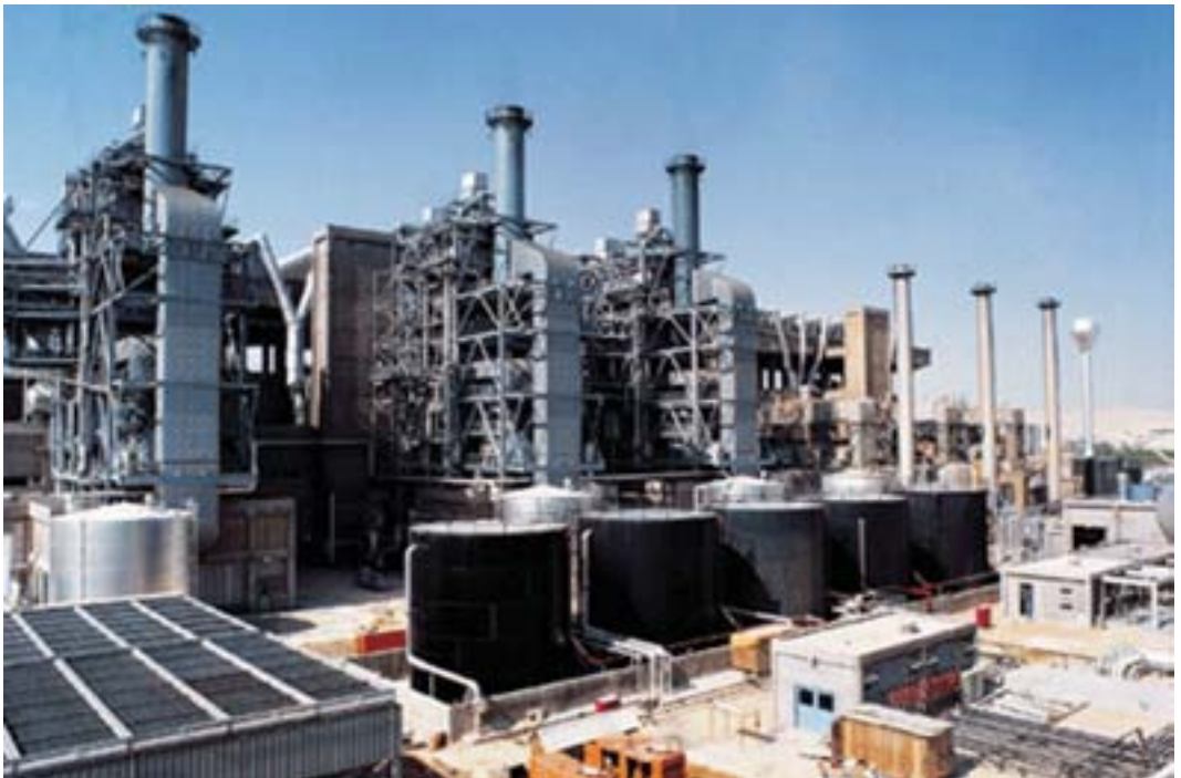
An overview of a thermal power station.
