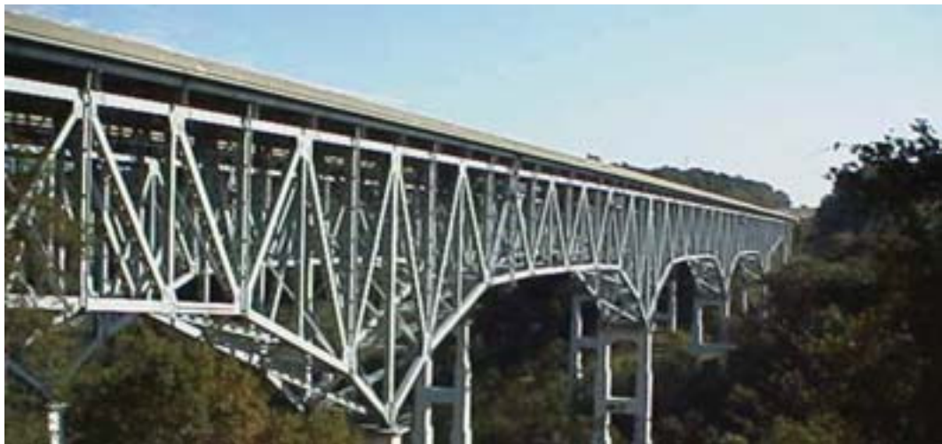
A railway bridge.
