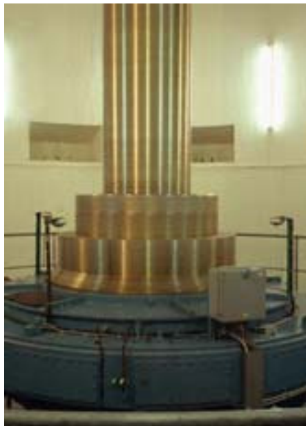
A big hydel generator. Governors are used to control the supply of working fluid (water in hydel generators).
