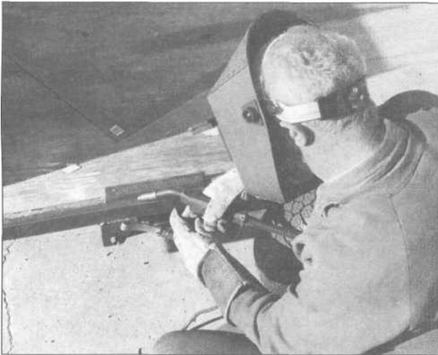
9.30 Short strips of 1/8-inch thick, 2-inch-wide strap metal (pre-drilled) were welded along the floor edges to help attach the bottom of the side panels. When MIG welding outdoors with argon gas shielding, use pieces of plywood around you to form a wind barrier to keep the gas from blowing away as you weld.
