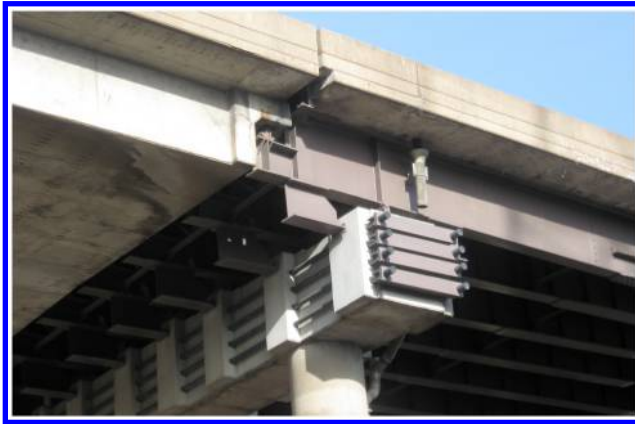
Figure 4. End condition between existing ramp and viaduct.
