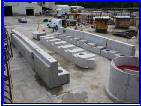
Figure 11. Substructure pre-assembly.
