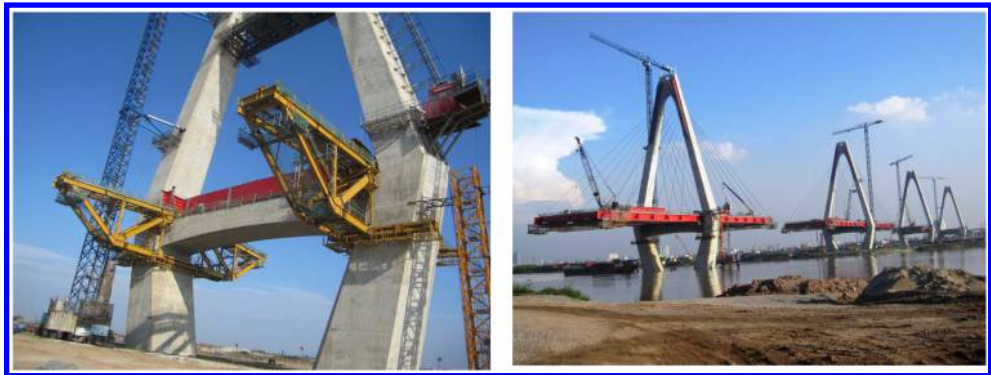
Figure 3. View of construction by inclined bent and cantilever erection.
