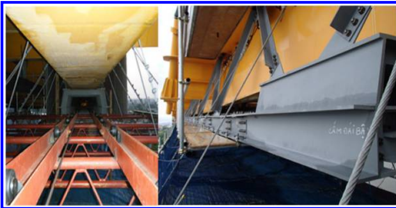
Figure 11. Temporary bypass truss.
