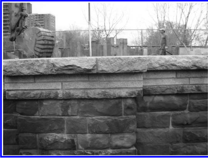
Figure 11. New Stone Coursing – delineation of original and raised profile, 2006.
