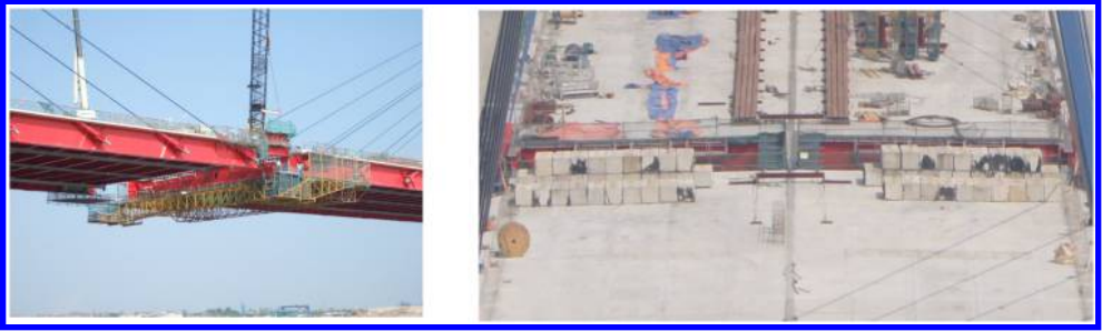
Figure 12. Closing work and counter weight concrete for closing work.
