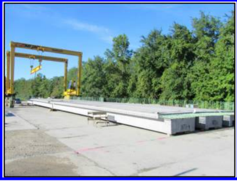
Figure 10. Superstructure pre-assembly.
