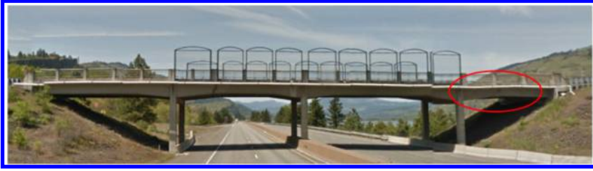
Figure 1. Mosier Bridge with highlighted Span 1 containing cracks at splice locations (Google Maps, 2014).
