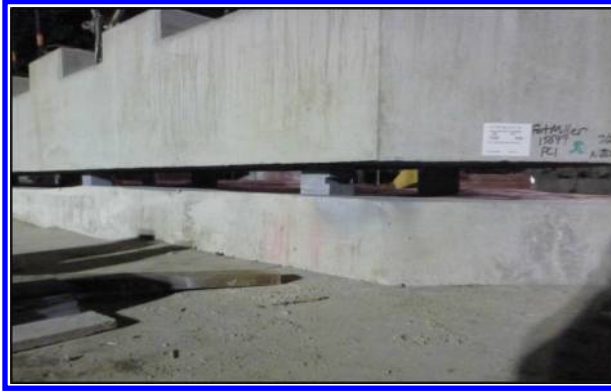
Figure 12. Precast unit on steel shims.
