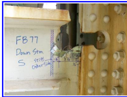
Figure 7. “Dog-bone” cutout retrofit with strain gages on lower deck FB 77 (PP 13).
