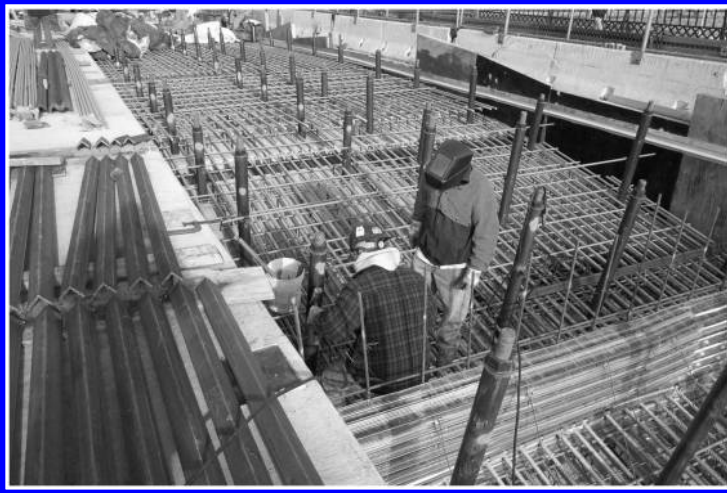
Figure 9. Setting Reinforcement Steel at Relief Arch, 2007.
