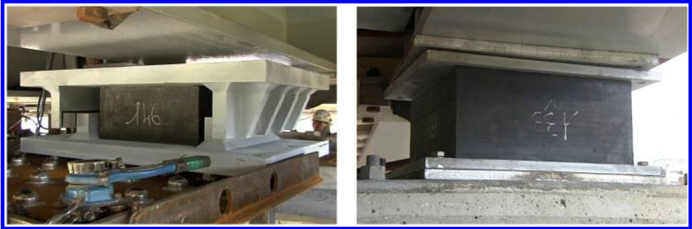
Figure 5. Lead rubber bearings installed in the bridge – guided (left) and multi-directional (right).
