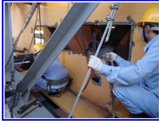
Figure 12. Cutting of Damaged part.
