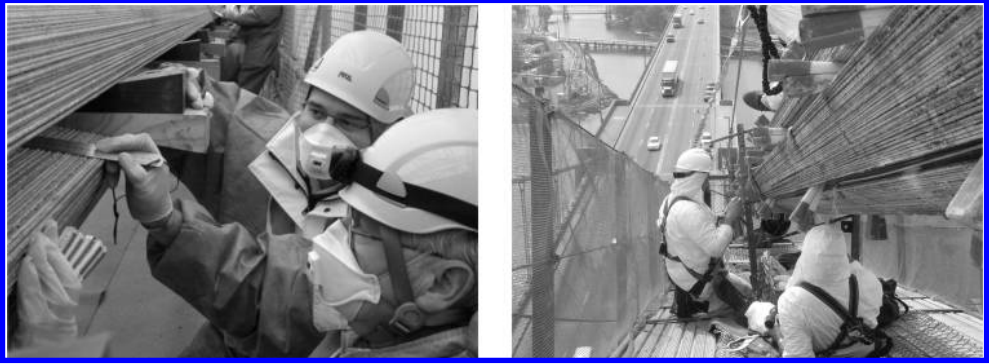
Figure 6. Internal cable investigation.
