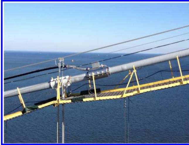
Figure 3. Injection sleeve and cable wrapping.
