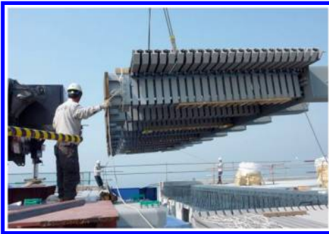
Figure 3. Installation of a Tensa-Modular expansion joint on a bridge with a concrete deck.
