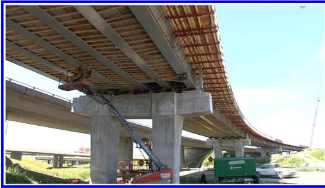
Figure 1. Construction of a curved highway viaduct.
