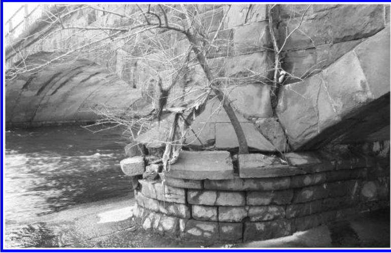
Figure 6. Existing Condition – Pier Nose, 2000.
