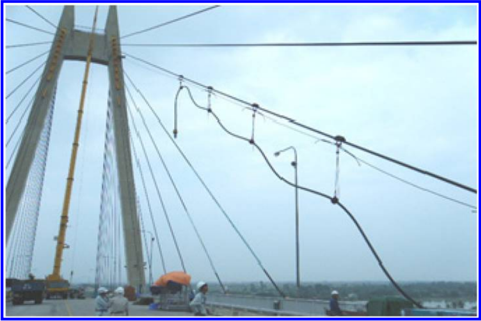
Figure 16. Dismantlement of stay cable.
