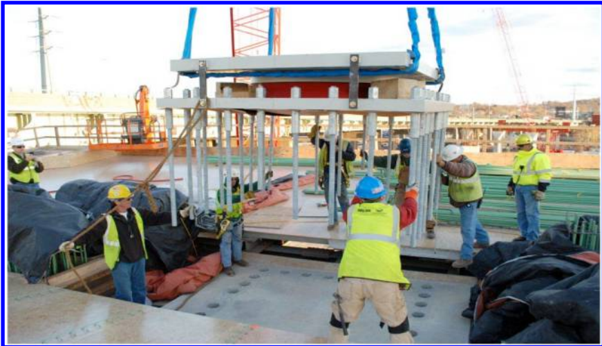
Figure 12. Disktron bearing installation at the Q Bridge.
