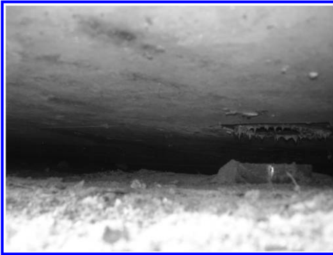
Figure 10. Deflection Gap between the Melan and Relief Arch, 2007.
