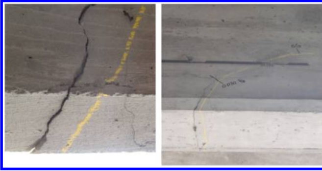
Figure 2. View of crack with vertical offset on interior girder of Span 1 (ODOT 2013).
