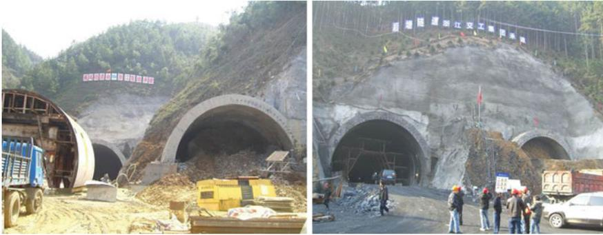
**Fig. 2.28** Field photos for excavation of small-clearance tunnels using pilot tunnel method
