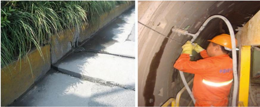
Fig. 5.4 Shield entry and re-filling of quick-hardening grout in the tunnel
