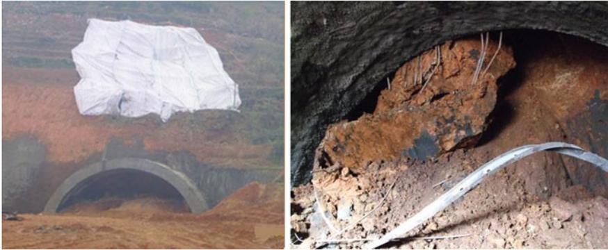
**Fig. 2.13** Tunnel collapse accident caused by supporting design parameters according to design code
