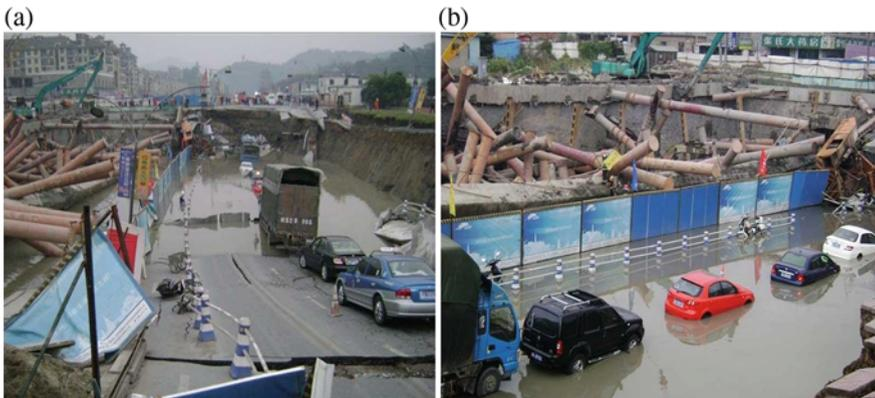
Fig. 6.4 Failure scene of deep foundation pit and support system
