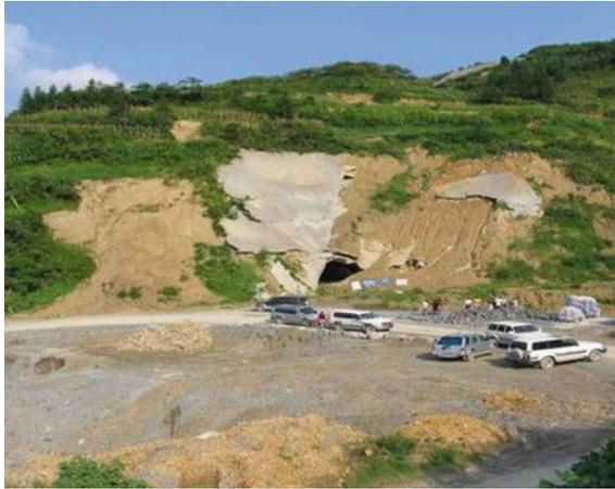
**Fig. 2.7** Surrounding rock failure caused by delayed supporting
