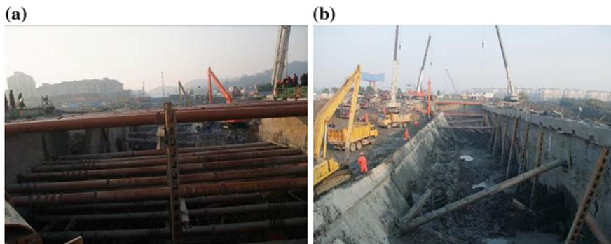
**Fig. 6.5** Support system before and after the Failure
