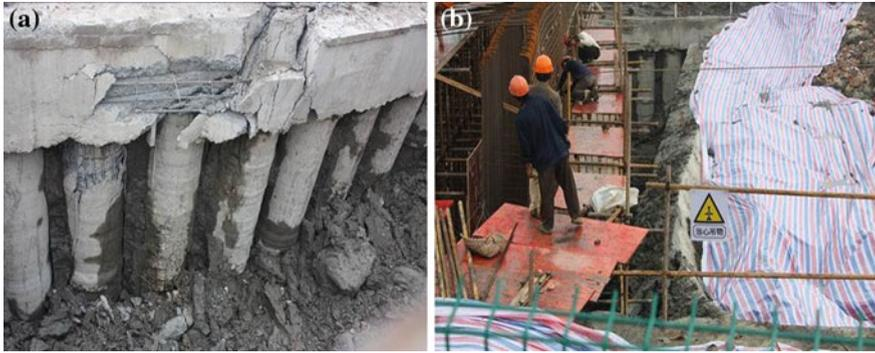
Fig. 6.3 Failure of foundation pit periphery beam and bored piles
