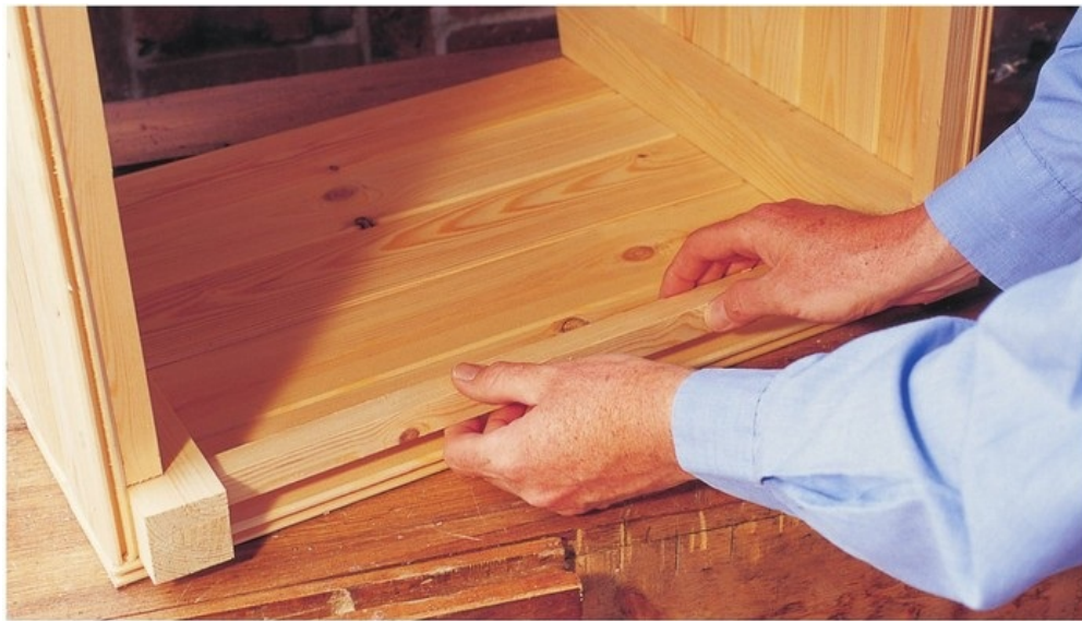
Fitting the support battens for the base panel.
