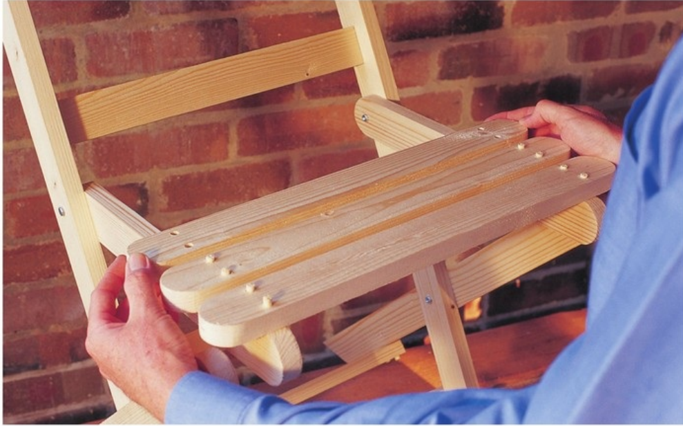
Seat slats are fastened to the seat rails with glue and dowels.
