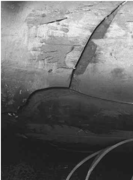
FIGURE 15.10 Cracks in three directions beneath the lagging.
