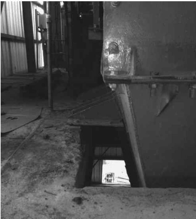
FIGURE 15.29 Hopper supported on the edge of the opening, possible failure during operation; recast and install (front view).
