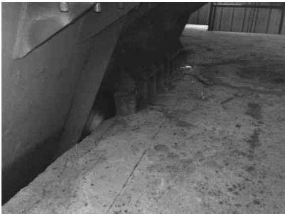
FIGURE 15.30 Hopper supported on the edge of the opening, possible failure during operation; recast and install (rear view).
