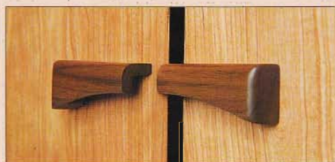
Handle detail showing rebate
