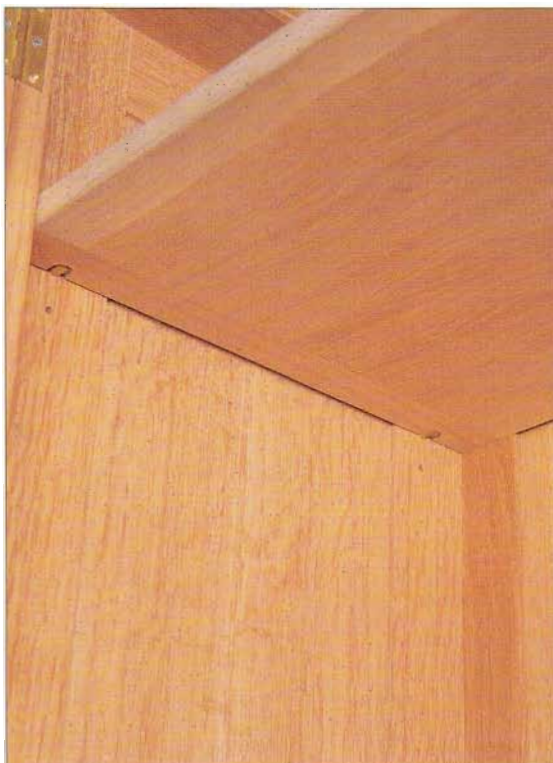
BELOW: Shelf is adjustable, supported on brass pegs
