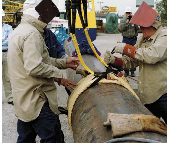
Illustration 11-1 – Induction Heating
