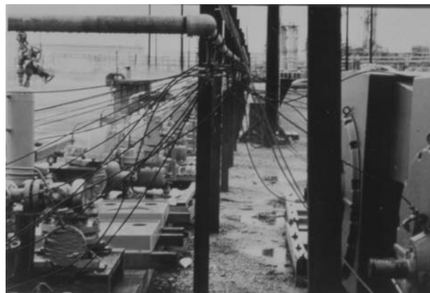
Figure 18-5. Temporary oil mist lines protect equipment prior to installation.
