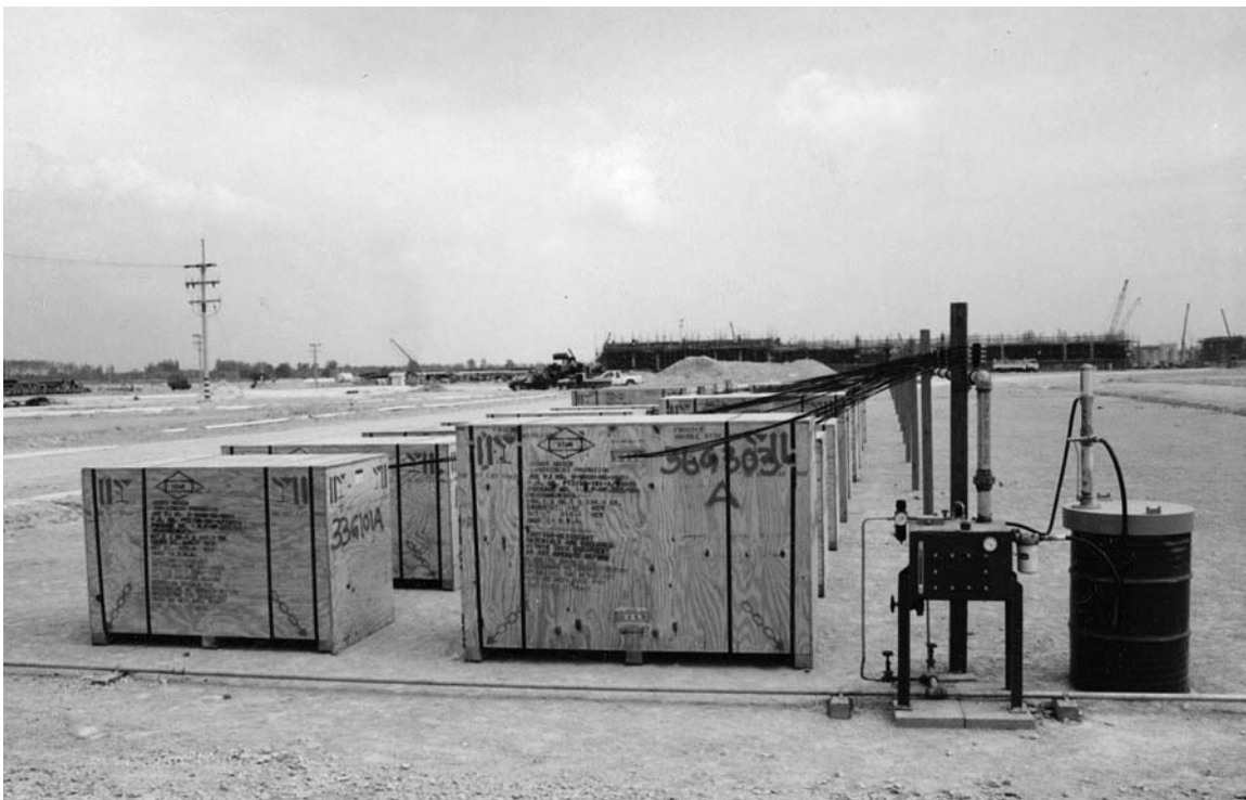
Figure 11-43. Outdoor storage of equipment before its installation at a grass-roots facility in Thailand (Source: Lubrication Systems Company, Houston, TX)
