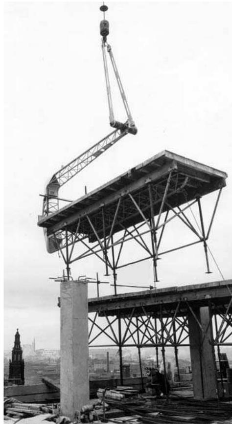
**Fig. 3.18** Crane handling a table form
