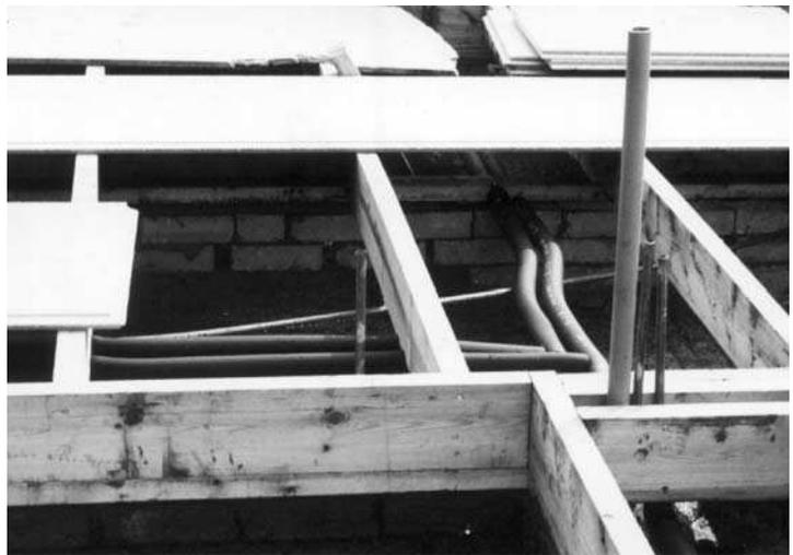
**Fig. 5.26** *Under-floor pipework*
