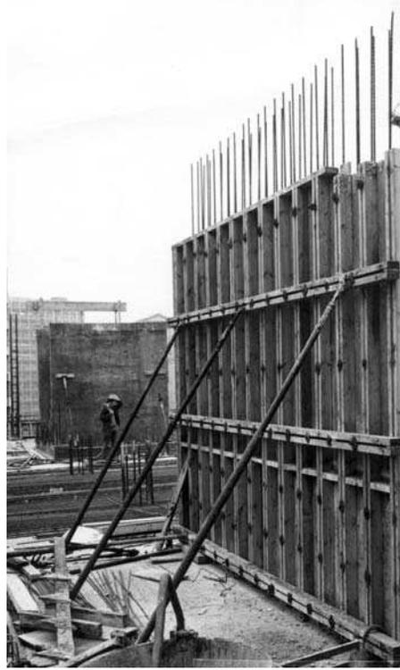
Fig. 3.13 Erection of wall form
