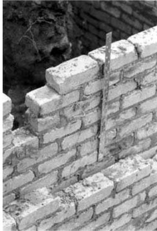
**Fig. 5.9** *Positioning holding-down straps*
