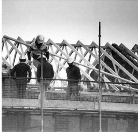
**Fig. 8.28** *Trussed-rafter roof being erected*
