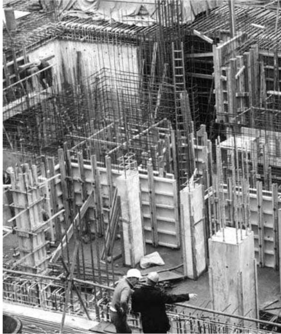
**Fig. 3.16** Formwork at different stages of construction
