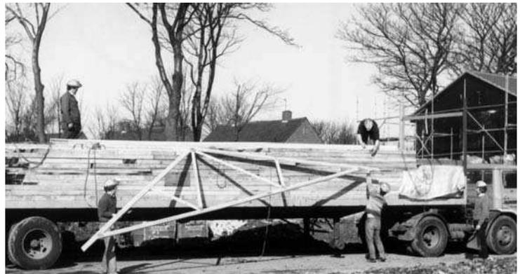
**Fig. 8.23** *Unloading trussed rafters*
