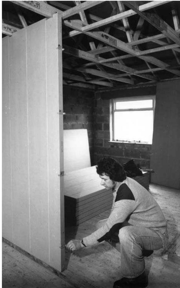
**Fig. 9.14** *Installing a 'Karpfos' partitioning system*
