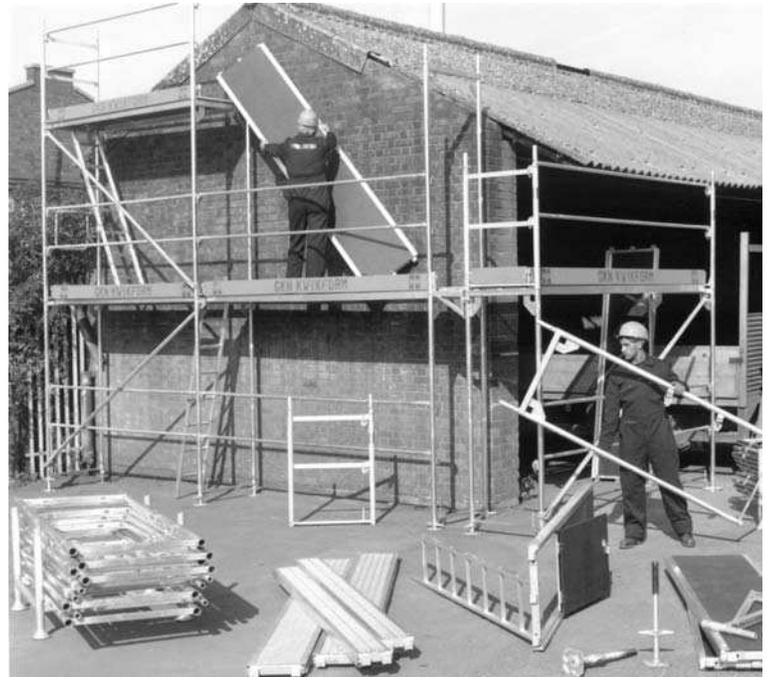
**Fig. 10.17** *Frame system scaffold*
