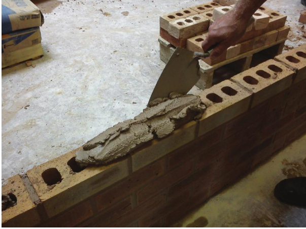
Fig. 111 Spreading mortar.
