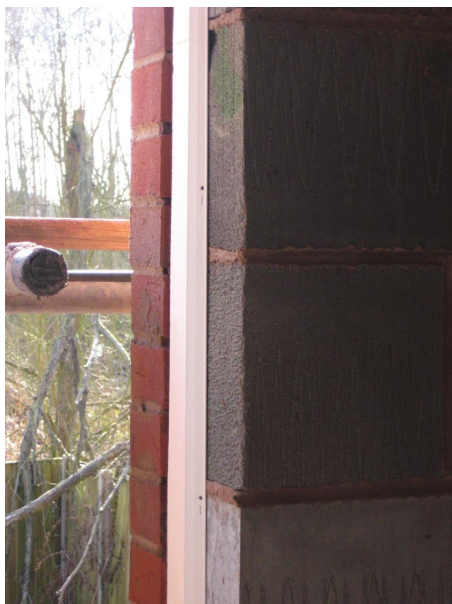
Fig. 184 Insulated cavity closer installed at a window reveal.
