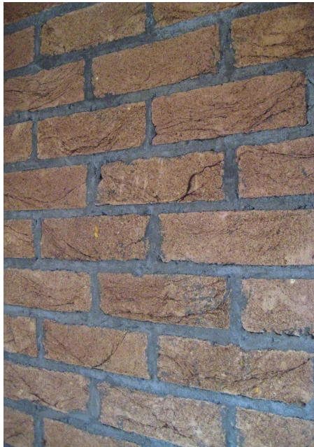
Fig. 163 Flush joint finish.
