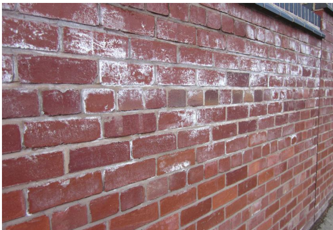
Fig. 264 Efflorescence.
