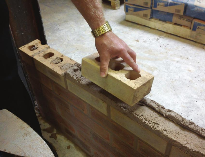
Fig. 114 The correct way to hold a brick.
