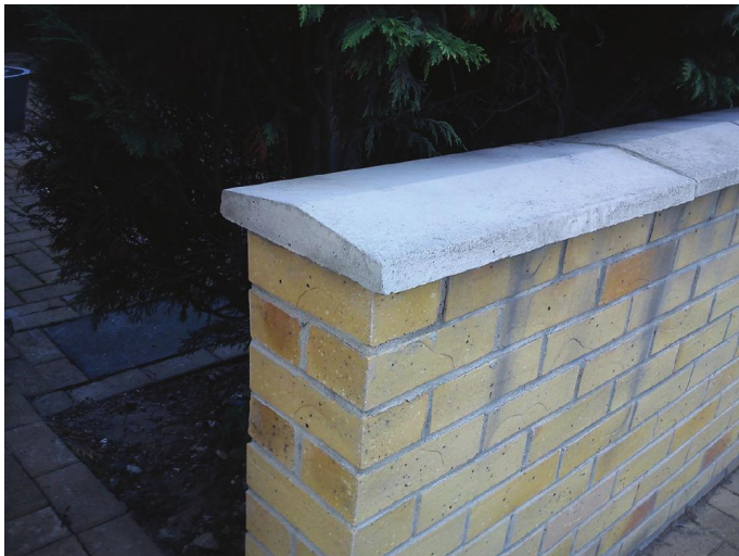
Fig. 242 Concrete coping extended to provide a weathering at a stopped-end.
