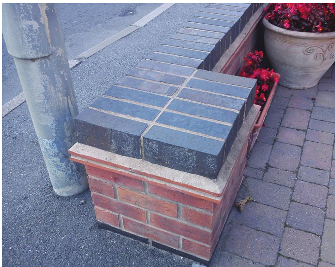
Fig. 235 Attached pier terminated at the same height as the wall.
