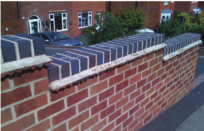
Fig. 227 Nibbed clay roofing tiles used as a single-course tile creasing.
