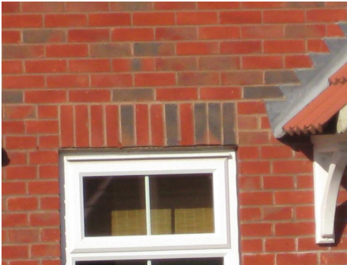
Fig. 254 Soldier course in a typical application, above a window opening.
