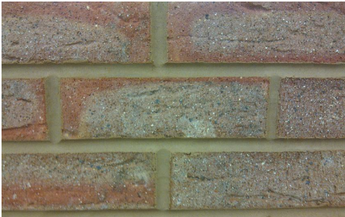
Fig. 154 Half-round joint finish.
