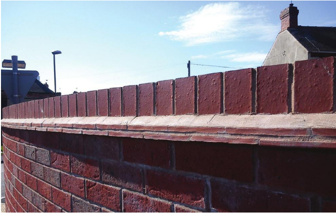
Fig. 226 Double-course tile creasing.
