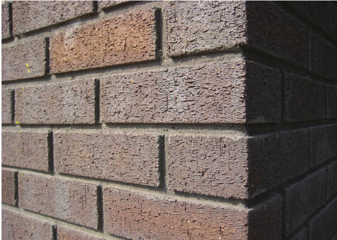
Fig. 157 Recessed joint finish.
