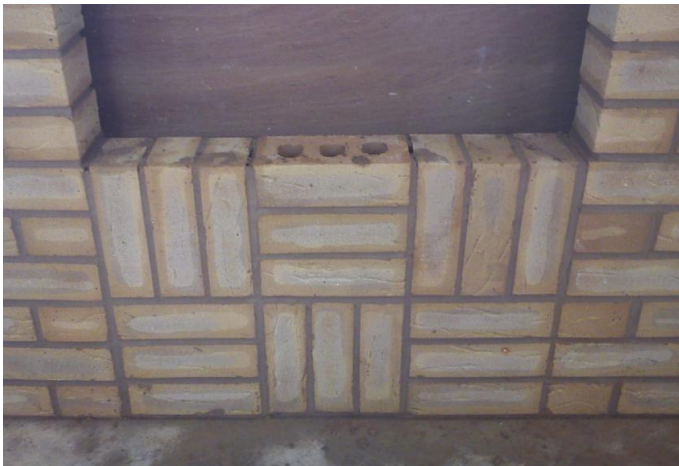
Fig. 258 Basketweave panel under construction within a pre-built square opening.
