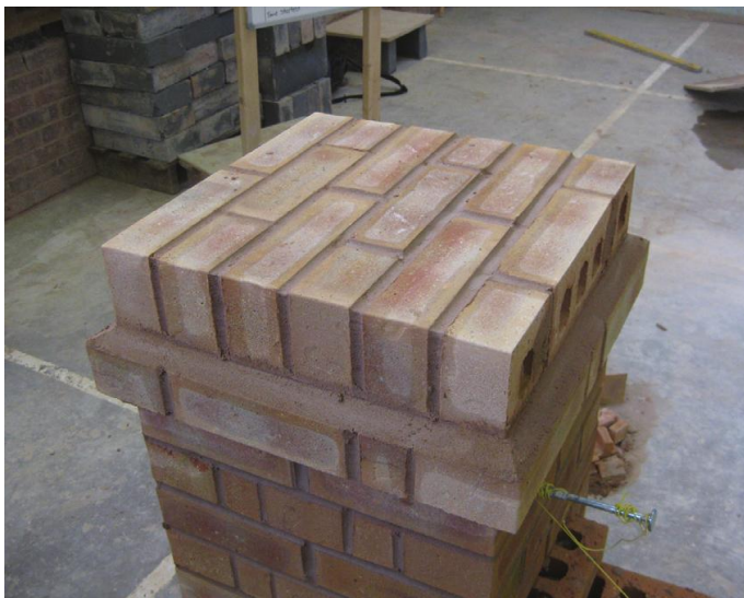
Fig. 237 Bonded brick-on-edge pier cap.
