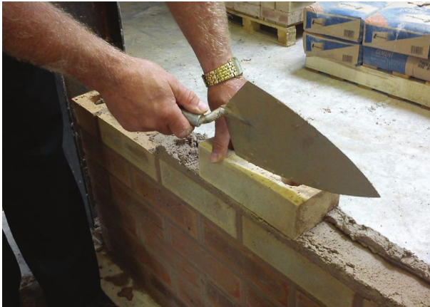
Fig. 115 Laying a brick.
