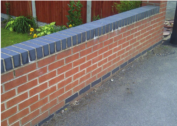
Fig. 208 Simple brick-on-edge coping using Staffordshire Blue engineering bricks.
