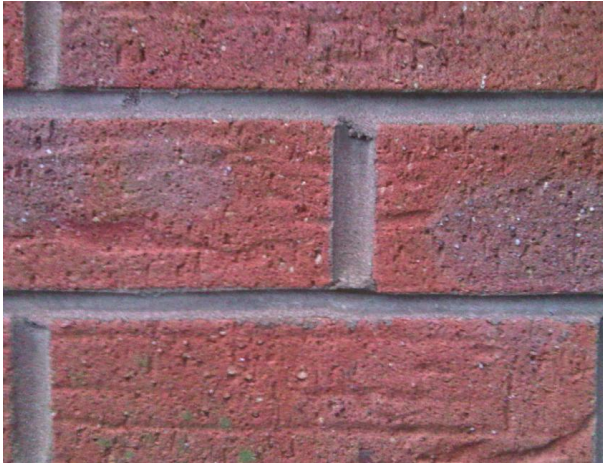
Fig. 156 Poor-quality half-round joint finish with 'misses' and poor 'topping and tailing' of cross-joints.
