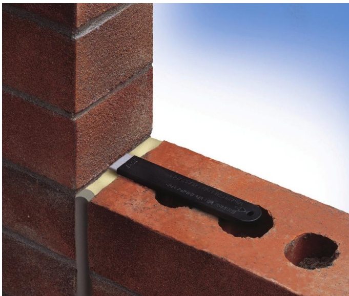
Fig. 244 Expansion joint with slip tie in situ. Ancon Building Products
