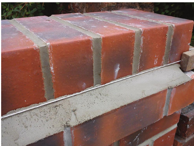
Fig. 231 Mortar fillet 'roughed-in' to the string-line.
