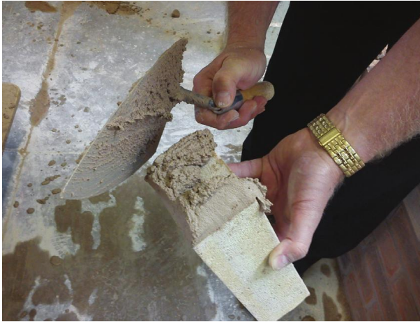
Fig. 120 Completing the cross-joint.
