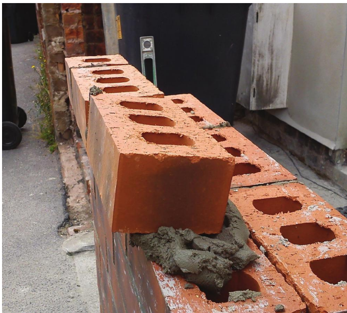
Fig. 221 Oversailing brick initially laid out of level, prior to adjustment.
