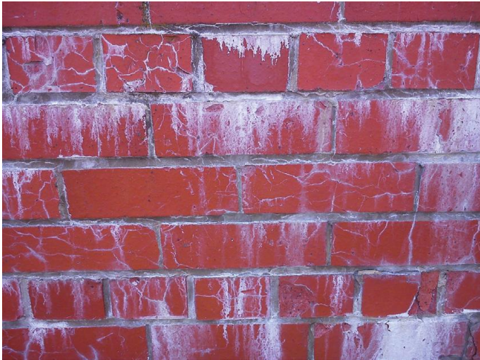
Fig. 265 Lime staining.
