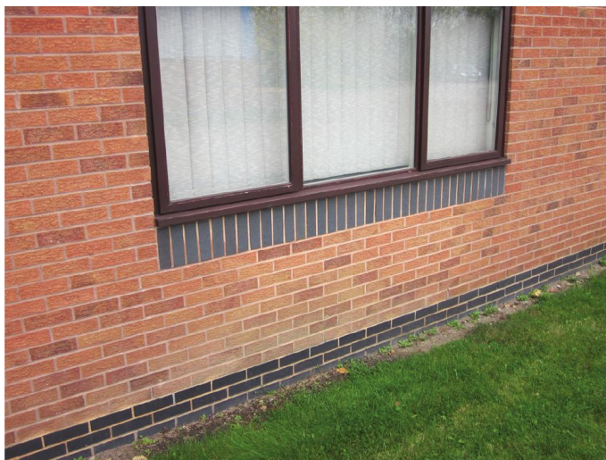
Fig. 256 Soldier course below a window opening at sill level.
