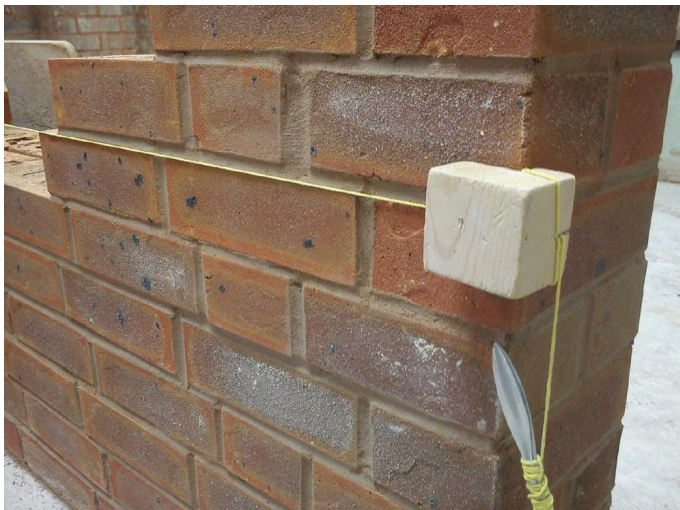
Fig. 135 Lines and corner blocks in use.
