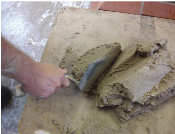
Fig. 107 Cutting mortar.
