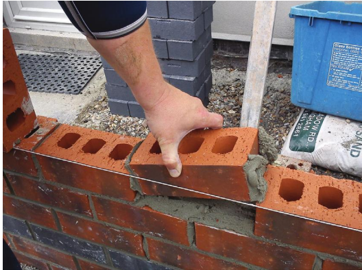
Fig. 141 Laying the last brick to a line.
