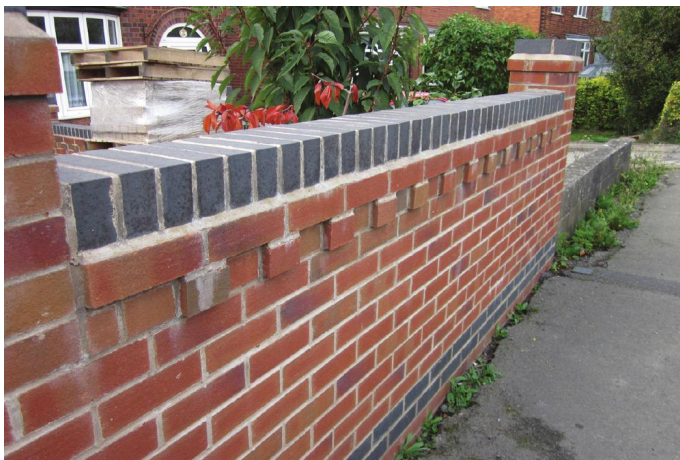
Fig. 252 Dentil course placed immediately beneath an oversailing course – a typical application, at the top of a boundary wall.
