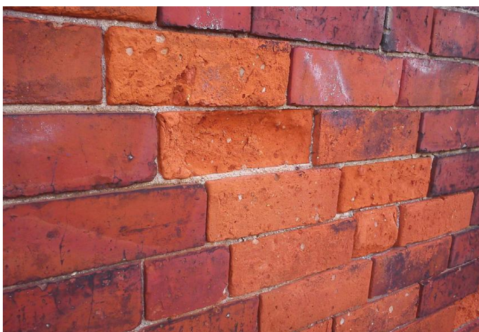
Fig. 267 Perished and spalled brickwork.
