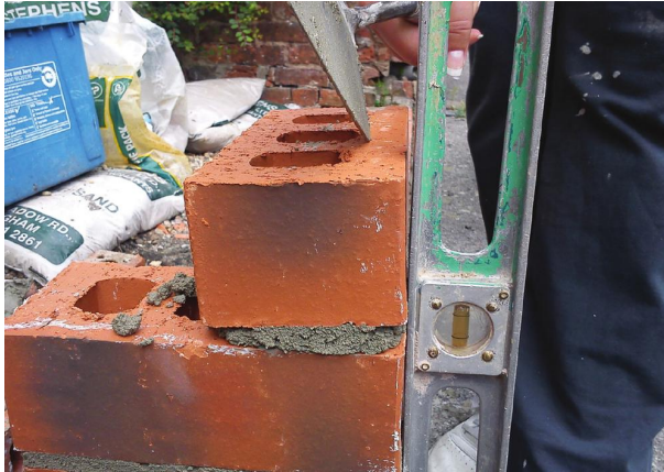
Fig. 130 A ligning the quoin brick to plumb.
