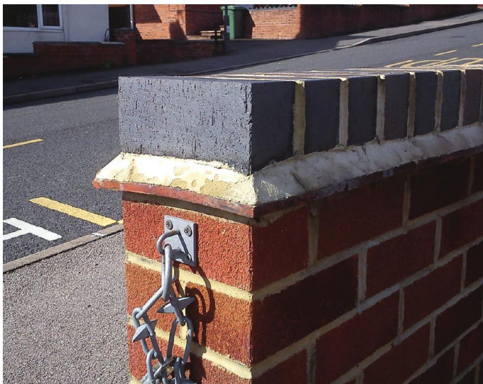
Fig. 229 Tile creasing extended to provide a weathering at a stopped-end.
