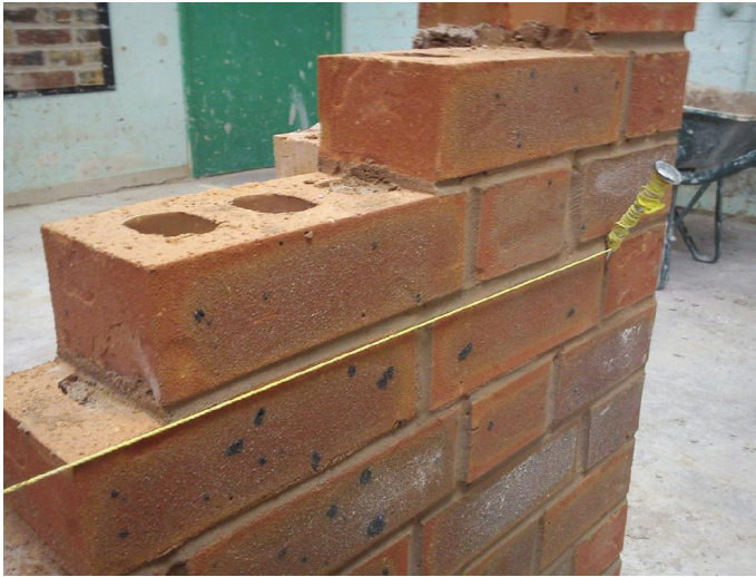
Fig. 134 Lines and pins in use.
