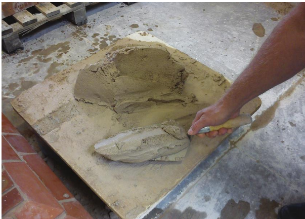
Fig. 110 Picking up the mortar.
