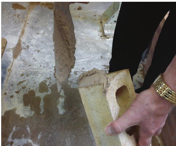
Fig. 118 Applying the first part of the crossjoint.
