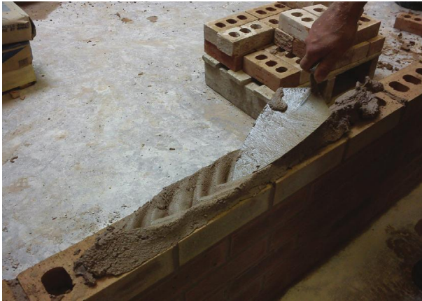
Fig. 113 Furrowing mortar.
