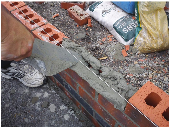
Fig. 140 Furrowing under the line.
