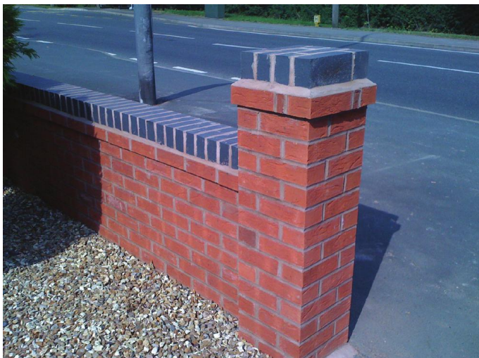
Fig. 236 Attached pier terminated higher than the wall.
