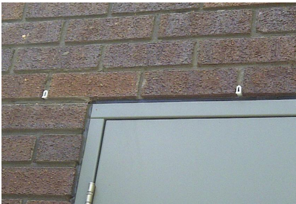
Fig. 191 Plastic weepholes inserted above a door opening.
