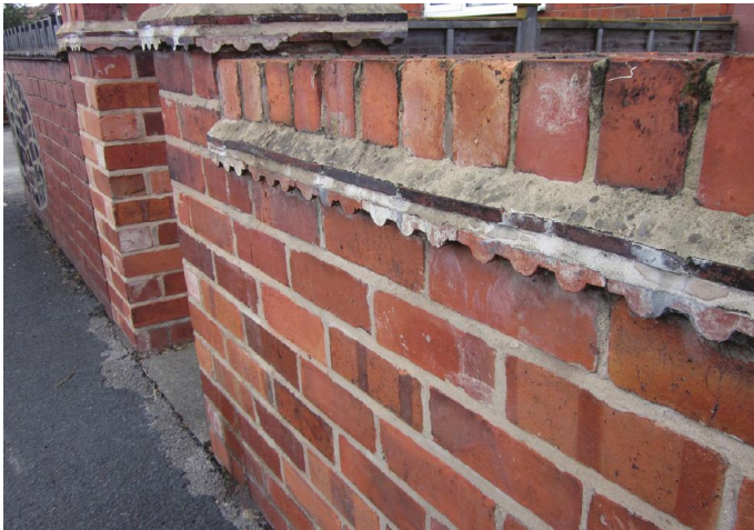
Fig. 228 Nibbed clay roofing tiles used as the lower course of a double-course tile creasing.
