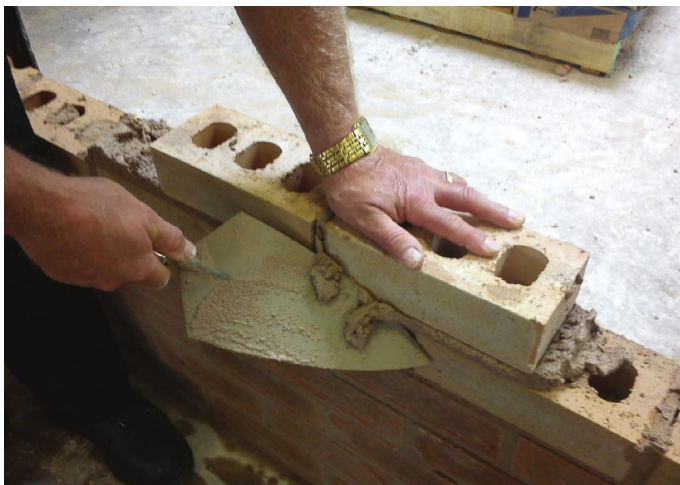
Fig. 121 Laying the next brick.
