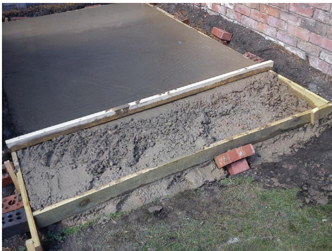
Fig. 47 Simple formwork for a small concrete base.
