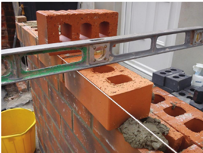
Fig. 222 All oversailing bricks must be checked for level across their width.
