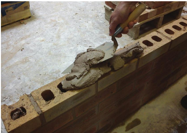
Fig. 112 Elongating the initial spread of mortar.
