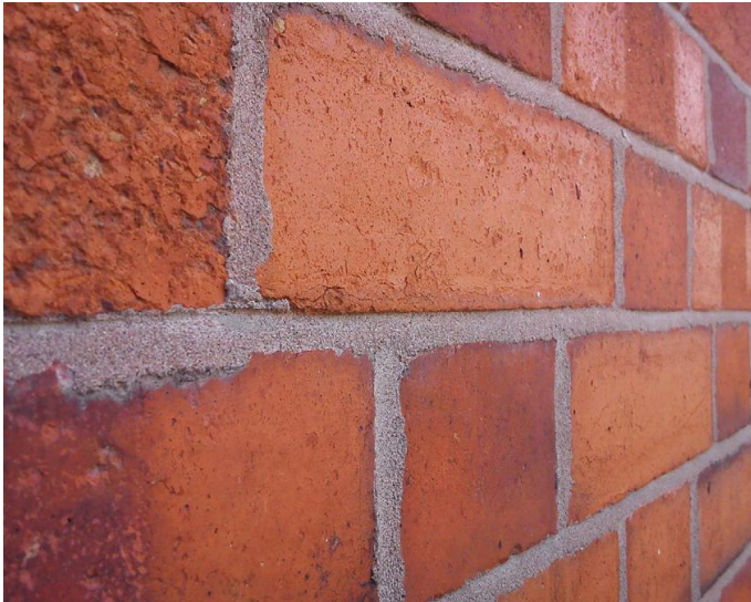
Fig. 161 Weather-struck joint finish.
