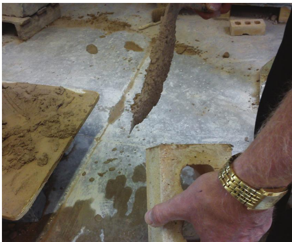
Fig. 117 Preparing to apply a cross-joint.
