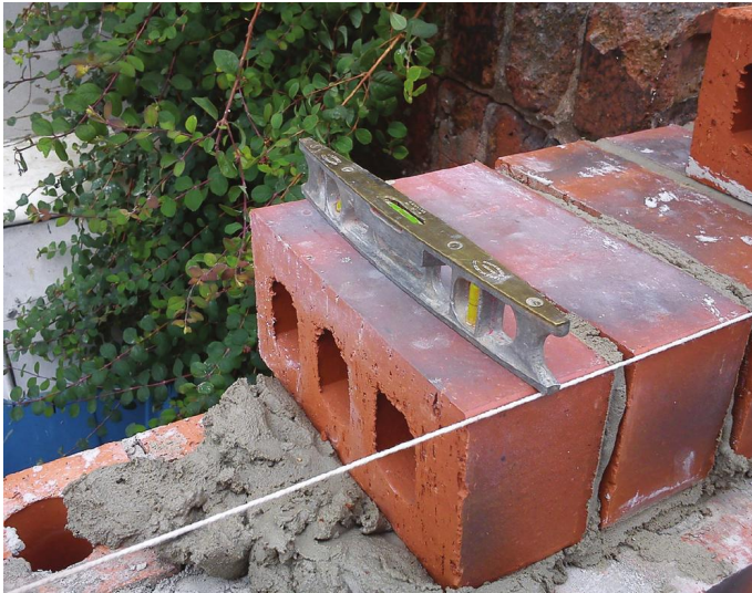
Fig. 212 Each brick-on-edge is laid to line and checked for level front to back.
