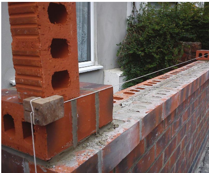
Fig. 210 Three bricks are laid at each end and a string line attached.
