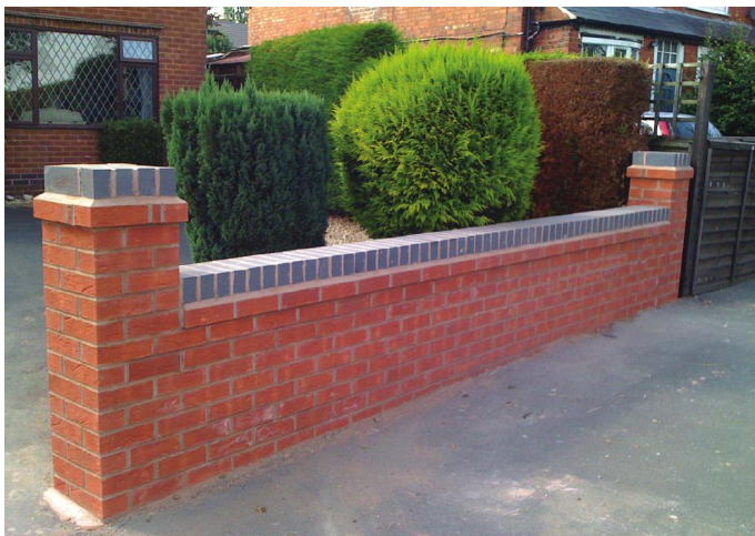
Fig. 218 Brick-on-edge coping laid on top of an oversailing course.
