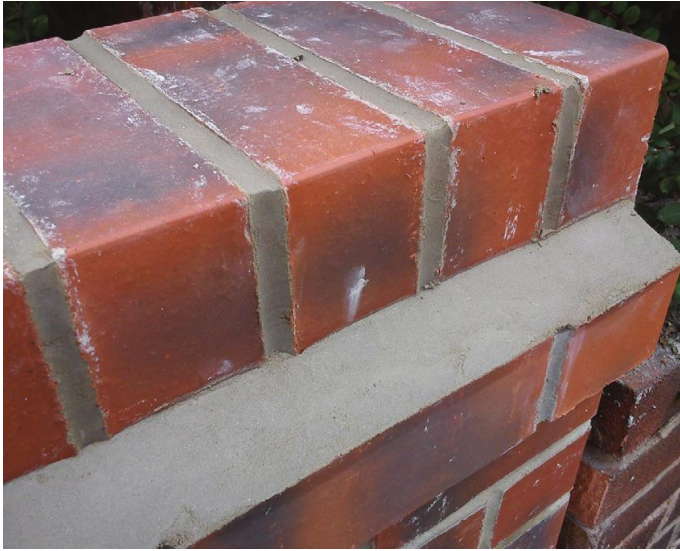
Fig. 233 Finished mortar fillet.
