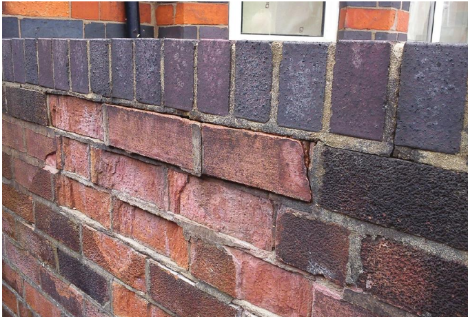
Fig. 217 Frost-damaged brickwork below a simple brick-on-edge coping.
