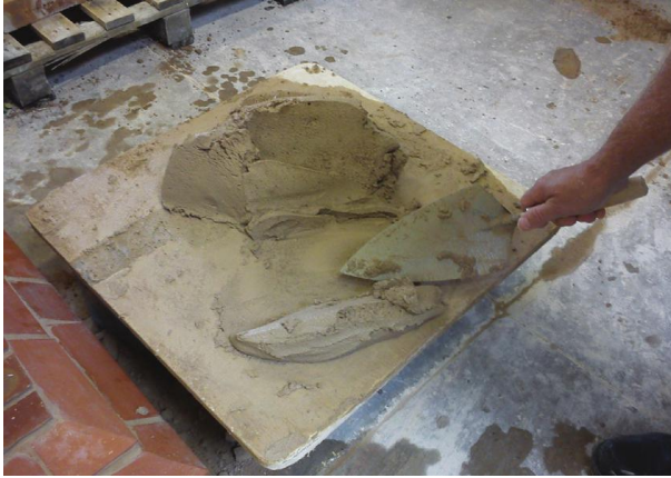
Fig. 109 Preparation for picking up the mortar.
