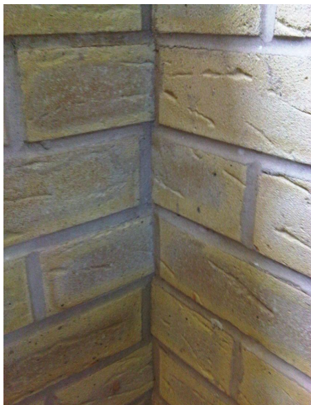
Fig. 165 Half-round jointing correctly finished at an internal corner.
