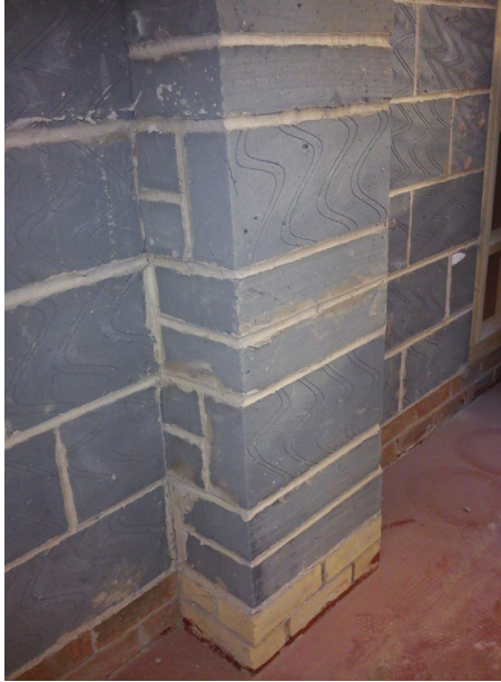
Fig. 104 Attached pier in blockwork.
