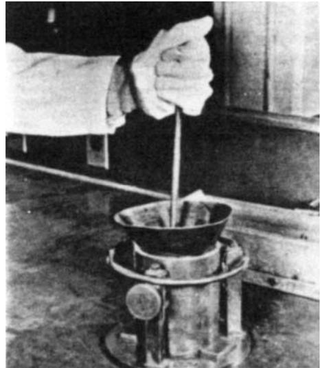
Figure 30 - Transferring the Mix to and rodding Mix in the Mold.
