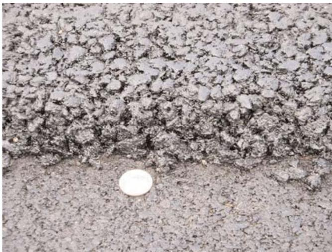
**Figure 2-6.** SMA surface course on dense-graded HMA base.
